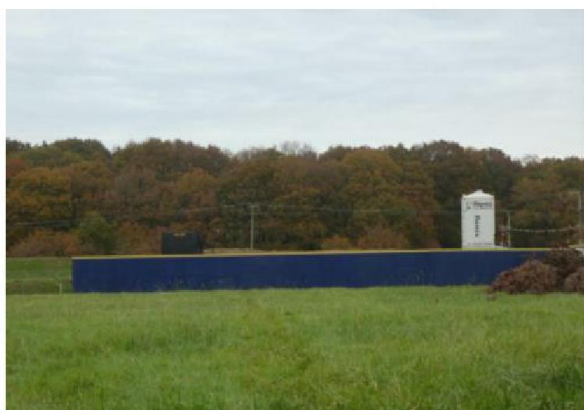
Photos of the spoil heaps on the site which were started in June 2024. By the middle of July they were over 60m long. Also the compound started in the summer of 2024 as shown in its completed state in November 2024.
