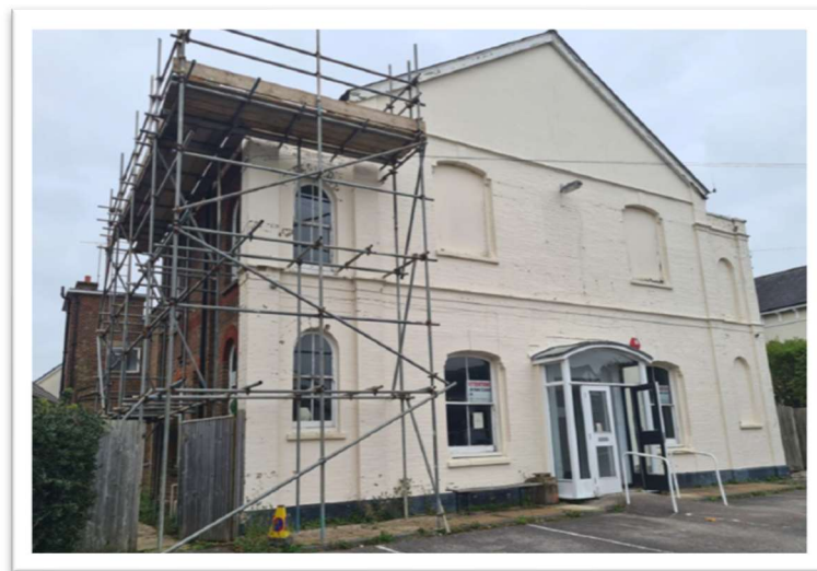
Image showing the current appearance of Park Centre
