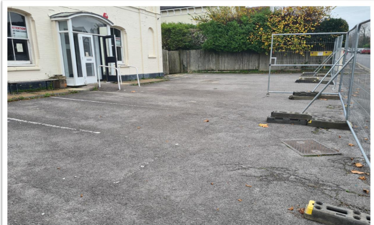
Plate 7.3: View across car park area to the front (south) of the building (looking north-east) – note the manhole indicating existing below ground services in this area
