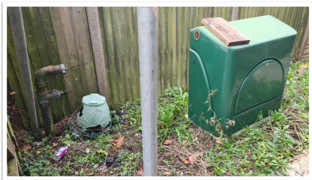
Plate 7.10: View of existing services to the west of the building
