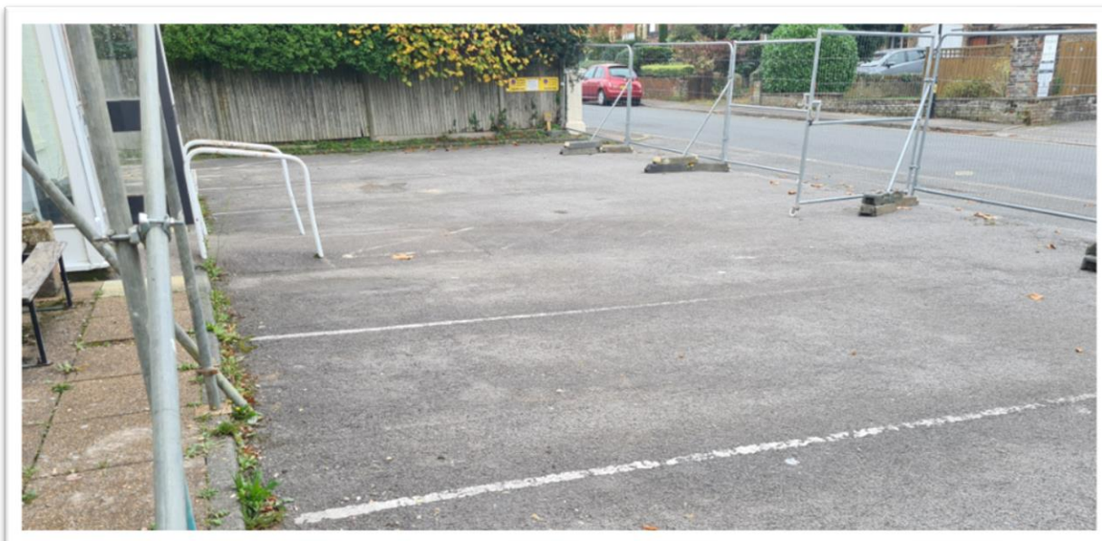
Plate 7.2: View across car park area to the front (south) of the building (looking south-east)
