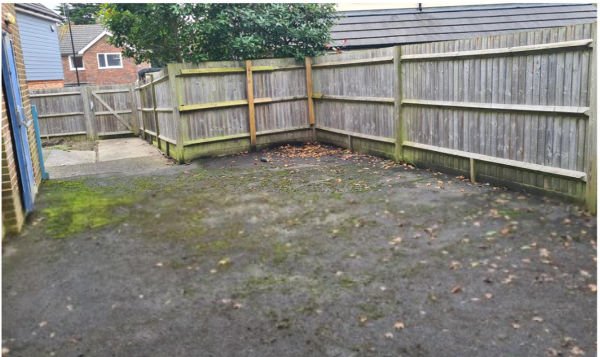
Plate 7.12: View of Tarmac area to the rear (north-east) of the building (looking north-west) – note the alignment of the culvert crosses the Tarmac area towards the gate along the western boundary
