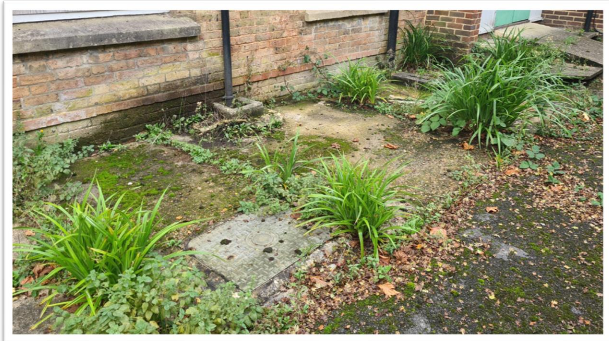
Plate 7.7: View of hardstanding areas and existing services in to the eastern side of the building where an extension is proposed
