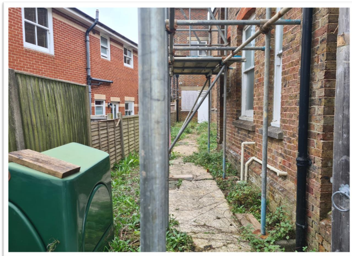
Plate 7.8: View of concrete path and area to the western side of the building where localised pad foundation and landscaping (paving) works are proposed (looking north)
