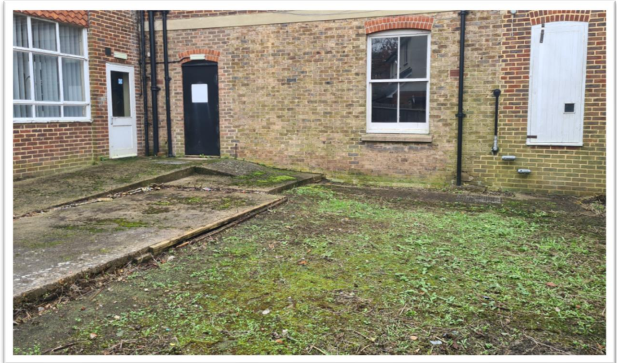
Plate 7.15: View of area to the rear (north-west) of the building (looking south) – note the various levels of concrete hard-landscaping – it is possible that some of this concrete is capping a below-ground feature, such as a soakaway or wartime shelter/bunker
