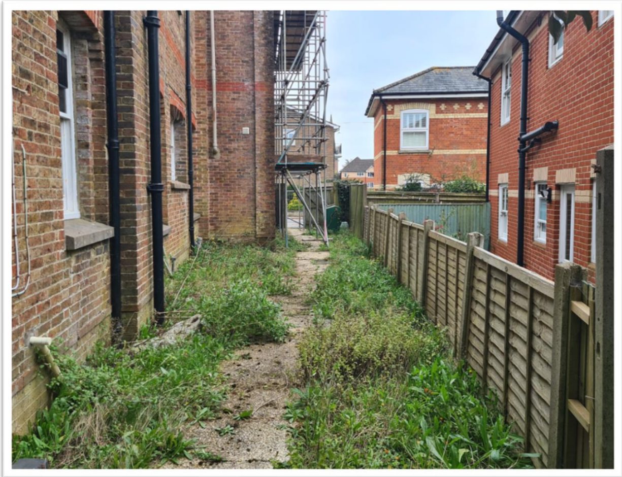
Plate 7.9: View of concrete path and area to the western side of the building where localised pad foundation and landscaping (paving) works are proposed (looking south)
