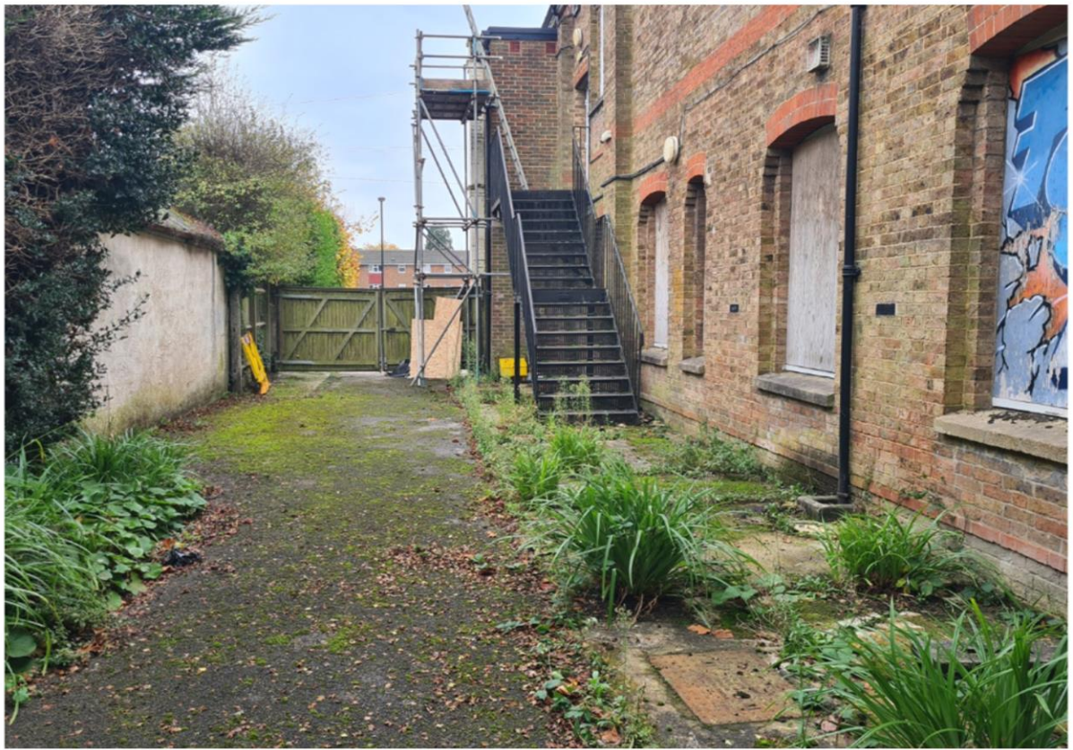
Plate 7.5: View of eastern side of the building where an extension is proposed (looking south)
