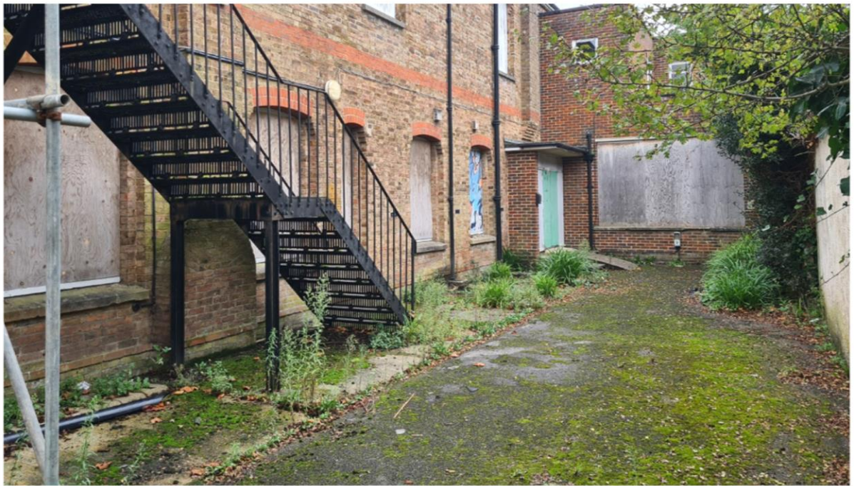
Plate 7.6: View of eastern side of the building where an extension is proposed (looking north)
