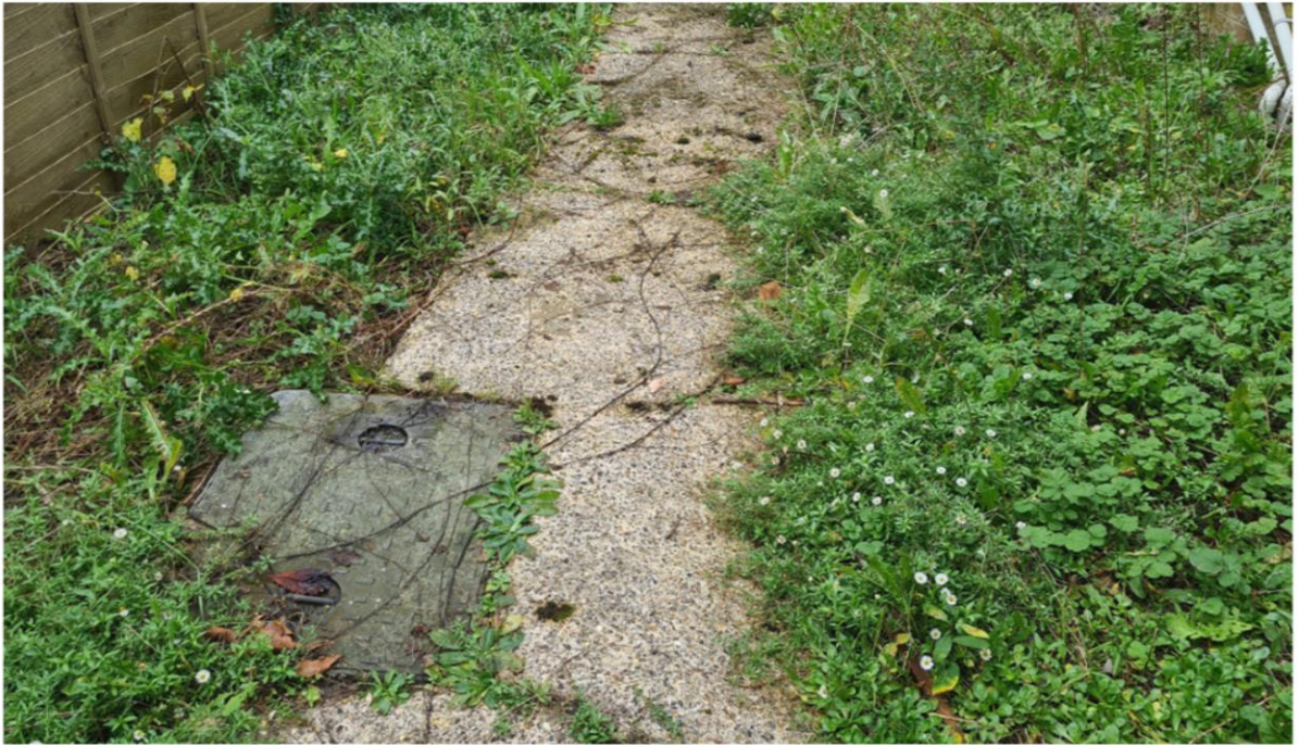
Plate 7.11: View of concrete path and existing below ground services to the western side of the building where localised pad foundation and landscaping (paving) works are proposed (looking north)
