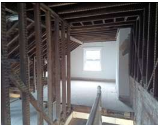
Photograph 11: The western elevation of the roof void in building B1.
