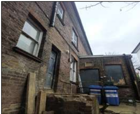
Photograph 3: Southern elevation of building B1.
