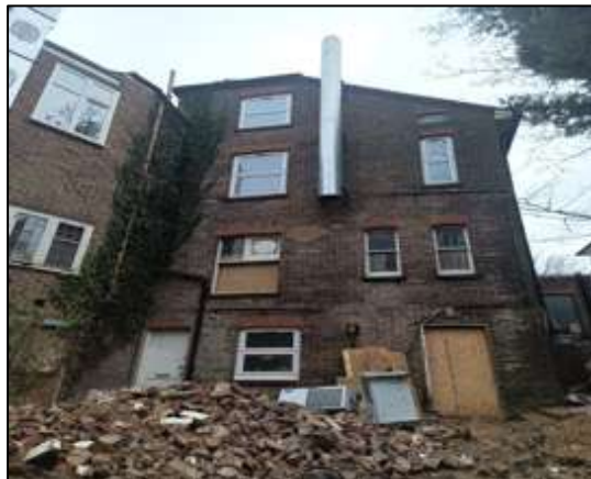
Photograph 4: Western elevation of building B1.
