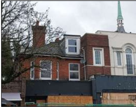
Photograph 1: Eastern elevation of building B1.
