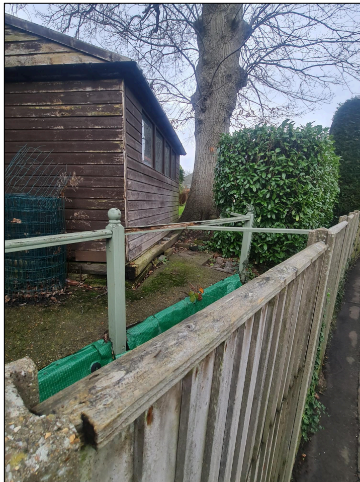
Figure 1: T3 viewed from the public footpath highlighting higher adjacent ground level.
