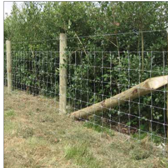
Western Boundary: Timber post and stock-proof fence (with rabbit proof base below ground)
