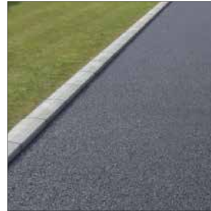
Access roads / paths: Tarmacadam surface.
