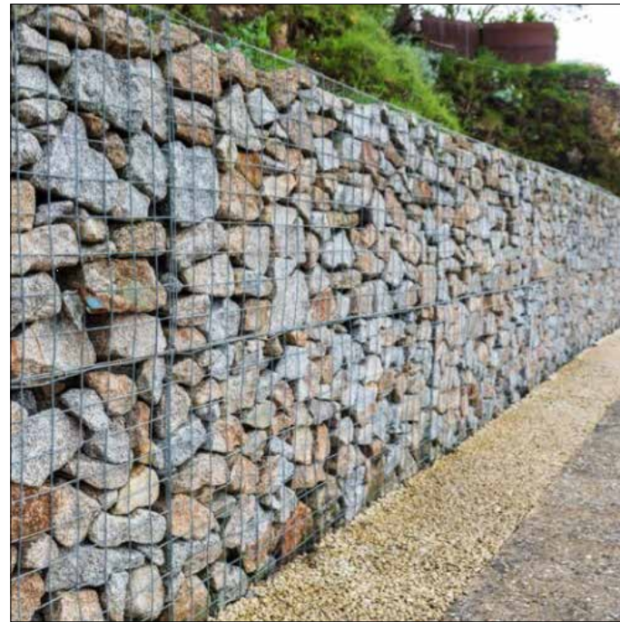
Retaining Features: Gabion Baskets.
