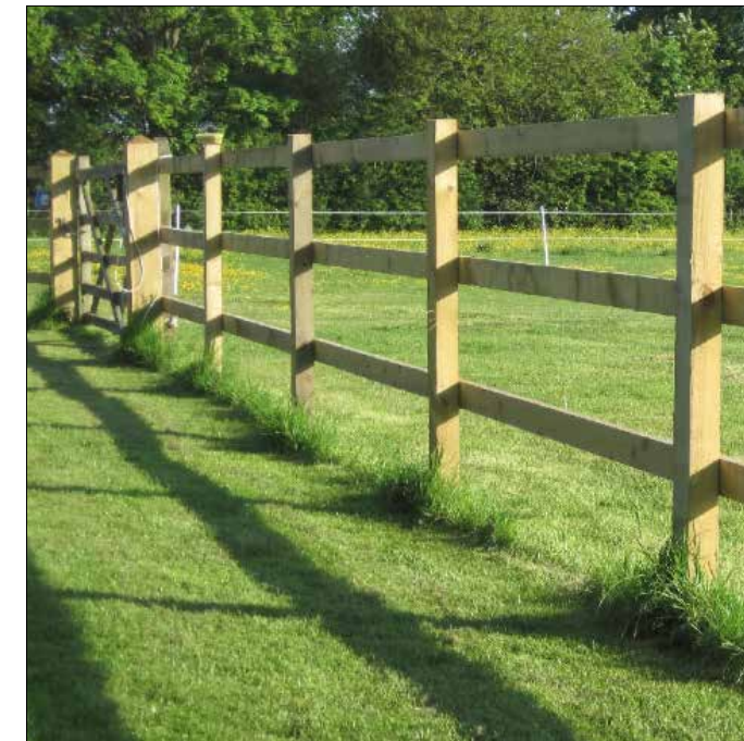
Edge Protection: Timber post and 3-rail fence.
