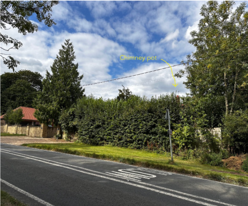
Approach entrance to site - existing two-storey house screened by existing vegetation.
