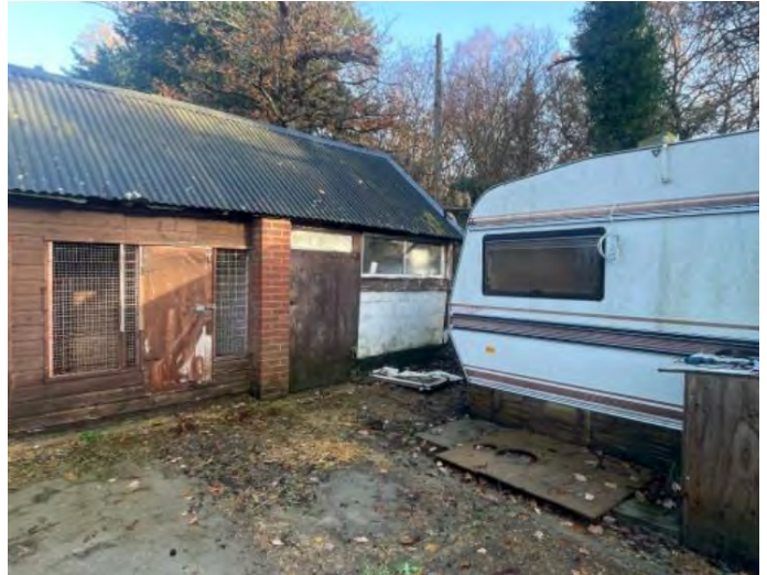
South eastern elevation of B2.
