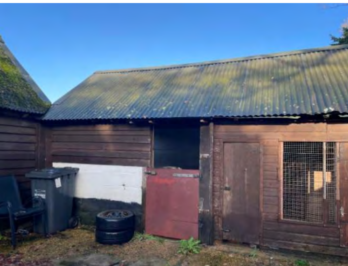
Open access into western section of B2.
