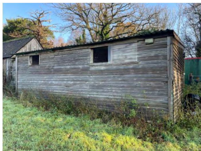
Western elevation of B6.
