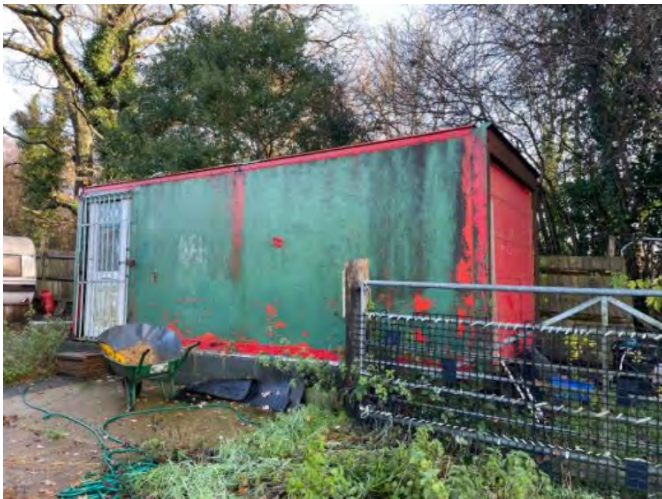
A static trailer with negligible suitability for roosting bats.
