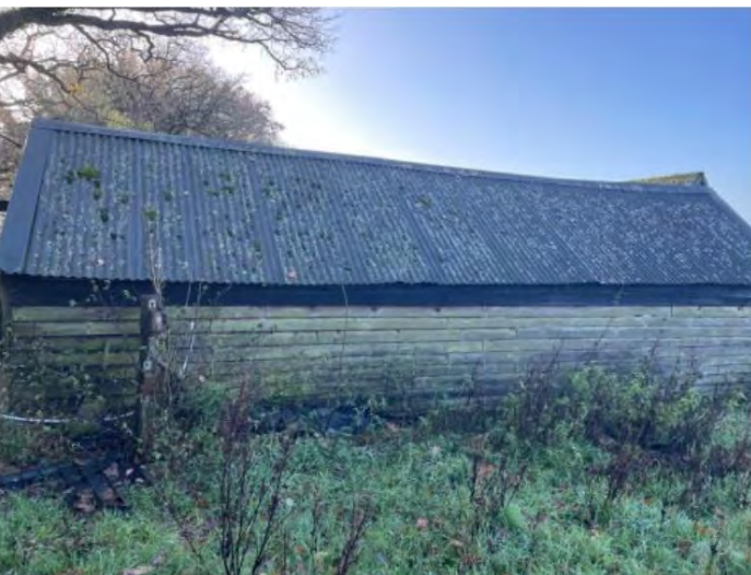
Northern elevation of B2
