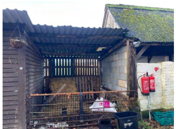
Hay store between B3 and B4 with no apparent bat roosting features.
