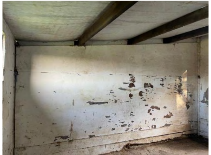
Interior of B6.
