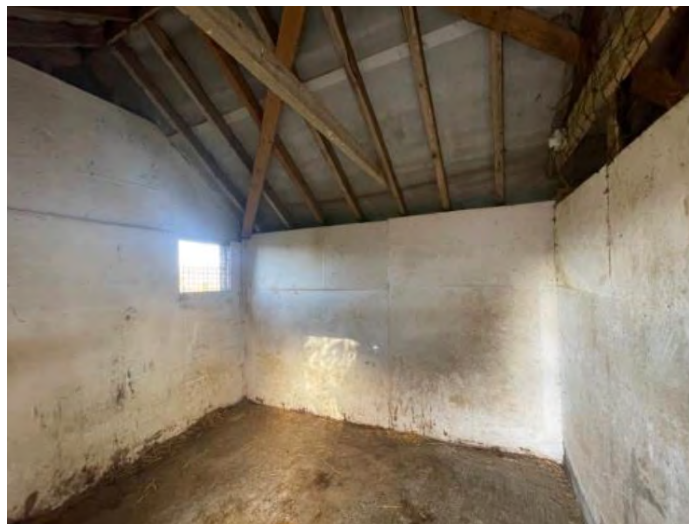
Interior of the western section of B2. The walls are lined, with potential crevice features between the lining and the exterior weatherboarding.
