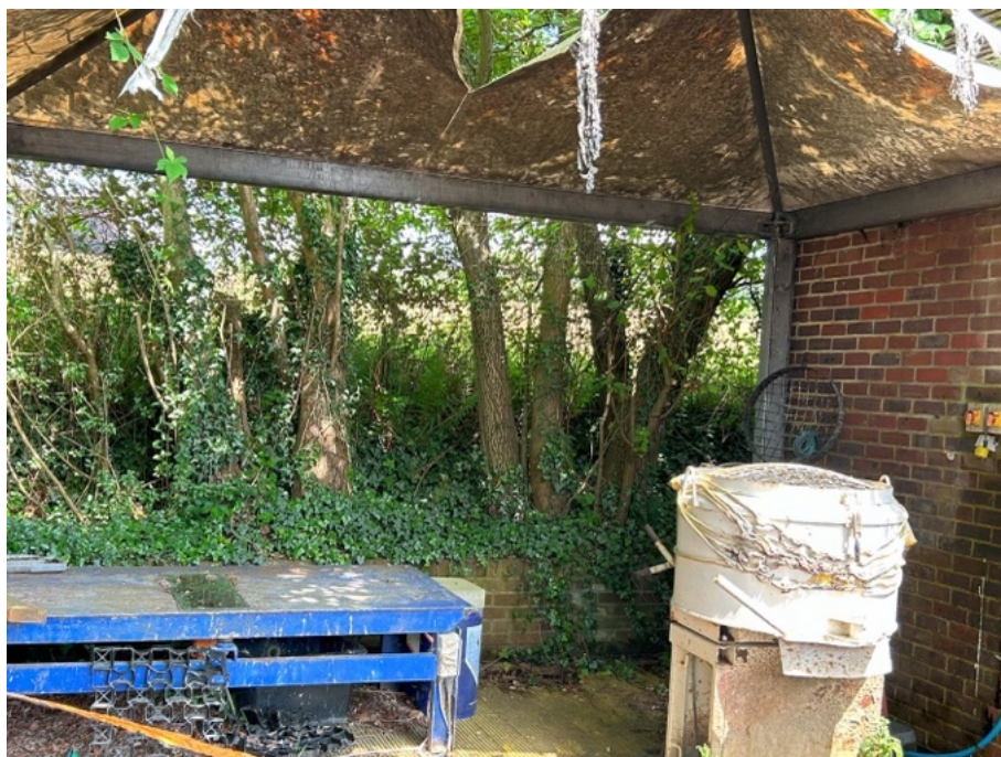
Image 6: Shows G41 – Goat willow group, rooted directly above retaining wall. They are to be removed to facilitate development as well as for arboricultural reasons
