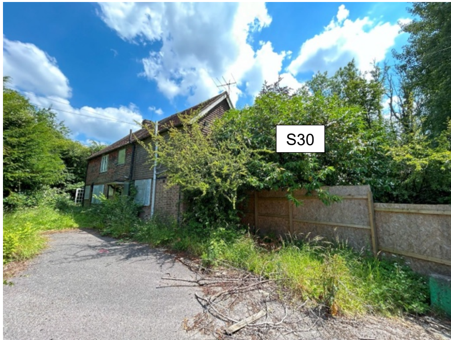
Image 5: Shows S30 – Laurel to be removed to facilitate works
