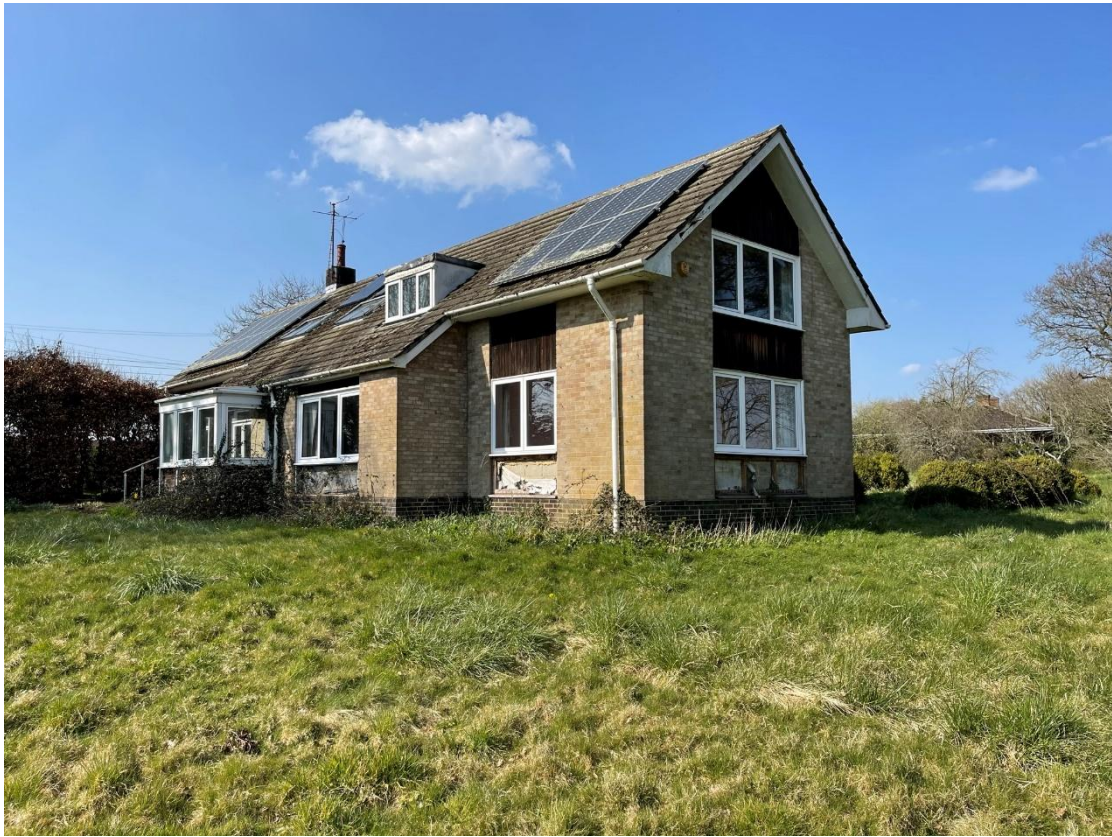
Image 01 – Showing the existing East Hookers Dwelling
