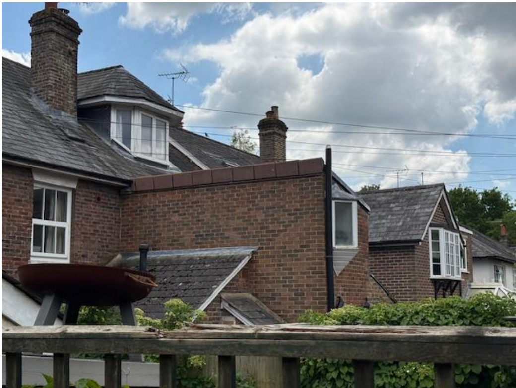
Rear view from 1 Francis Road towards Number 3,4,5 & 6 Francis Road
