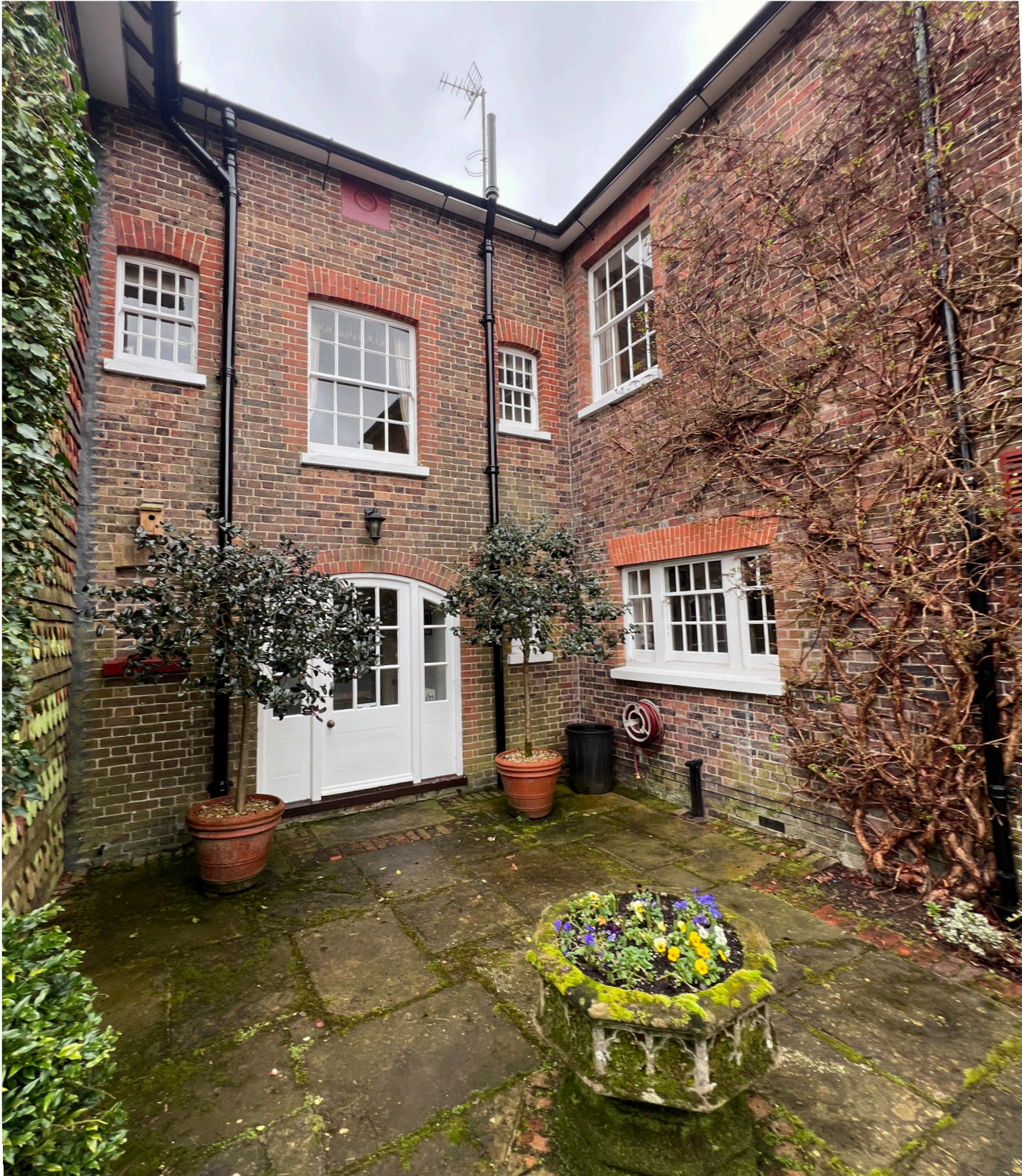
Rear courtyard formed between the eastern and western wings of Sunte House
