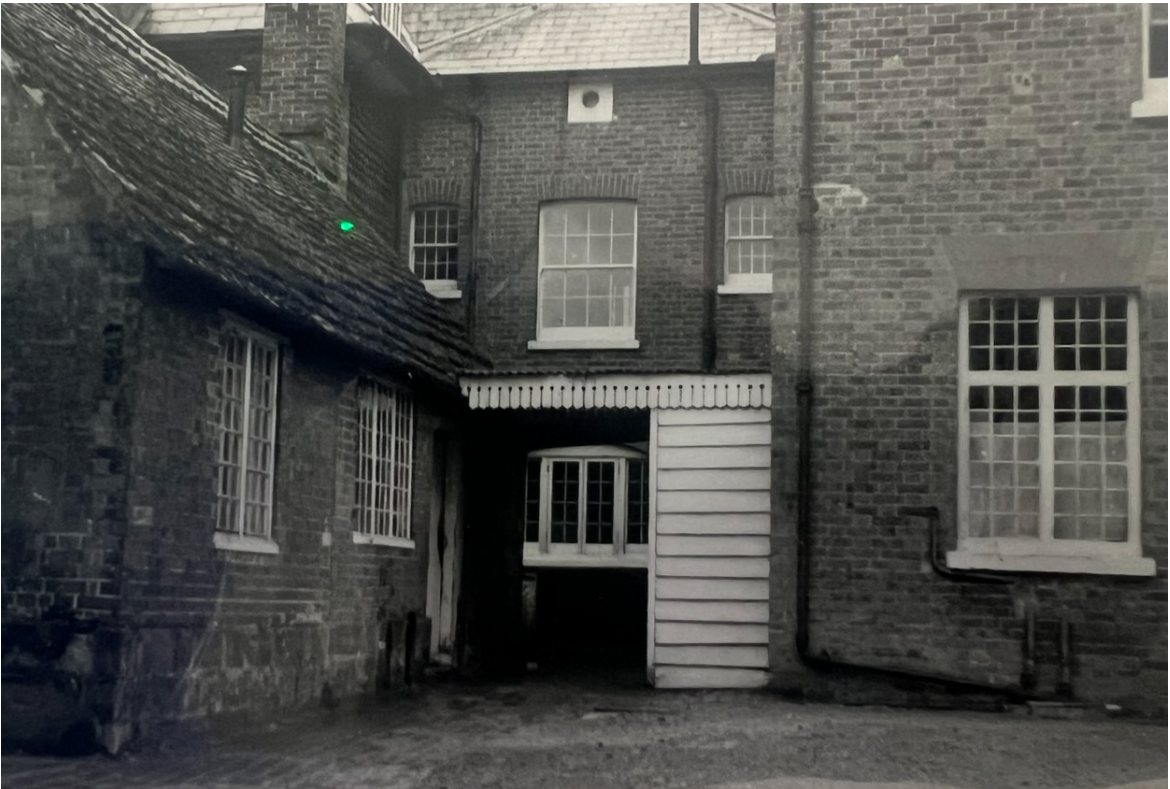
Former extent of The Dairy and canopy link before their demolition was approved under listed building consent HH/013/88/LBC
