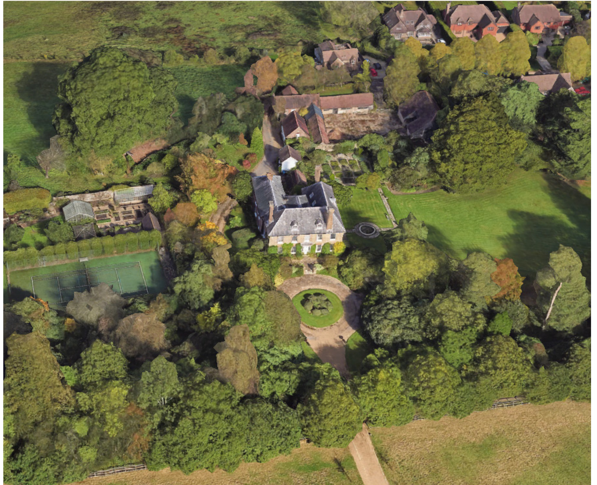
Sunte House and associated buildings, set within a part rural, part suburban context (Google Earth)
