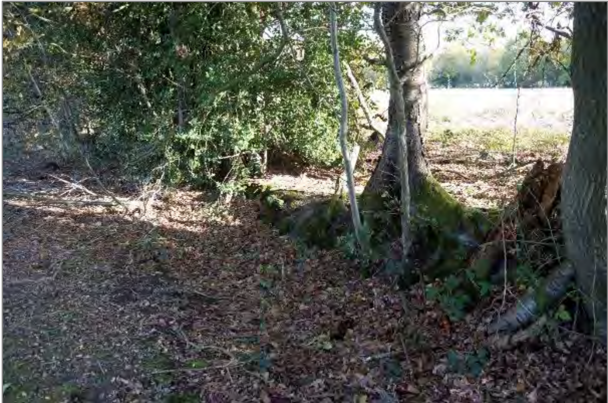
Plate 12: (Silted) Ditch and bank boundary typical of those dividing the site
