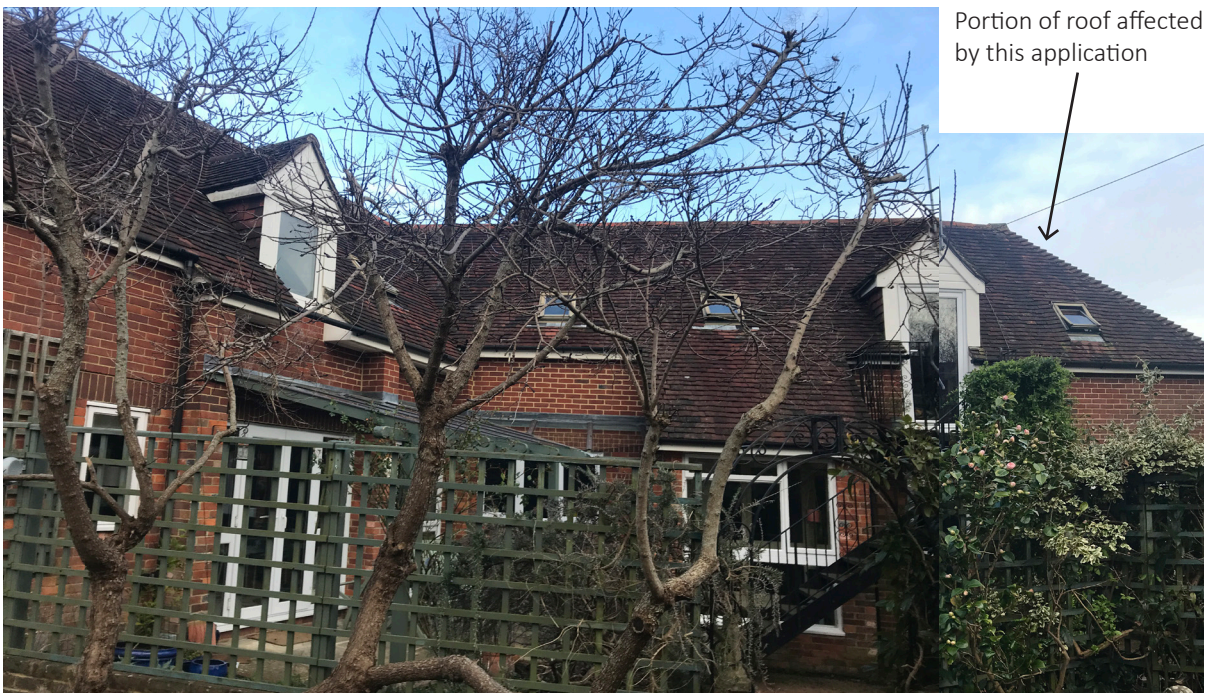
The roof where alterations are proposed under this application is not visible from the street
