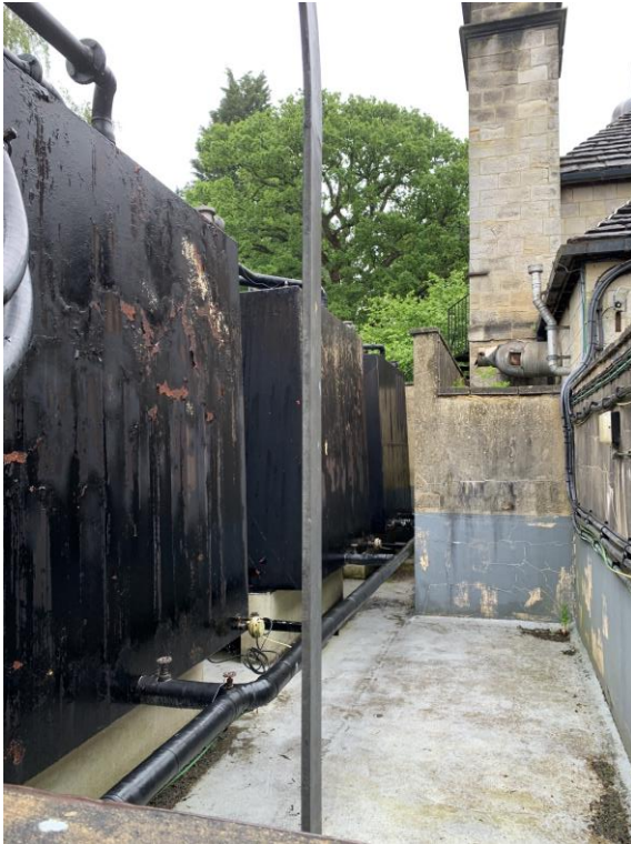
Photos showing location of three external oil tanks and two internal oil-fired boilers on concrete plinths.
