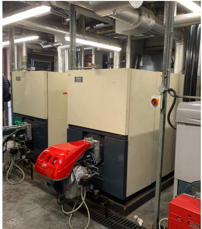
Photos showing location of three external oil tanks and two internal oil-fired boilers on concrete plinths.
