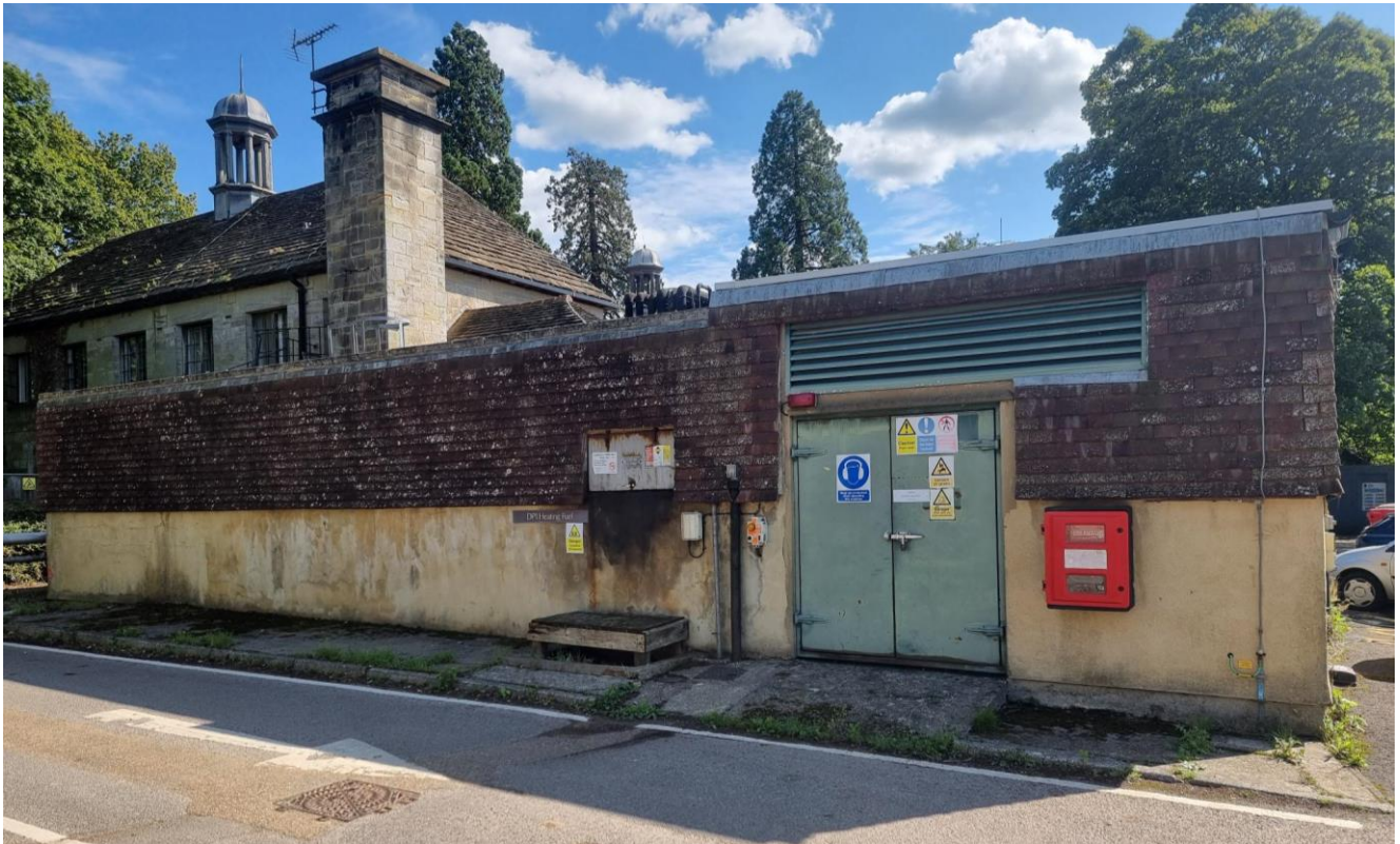
View of the northern wall of the compound.
