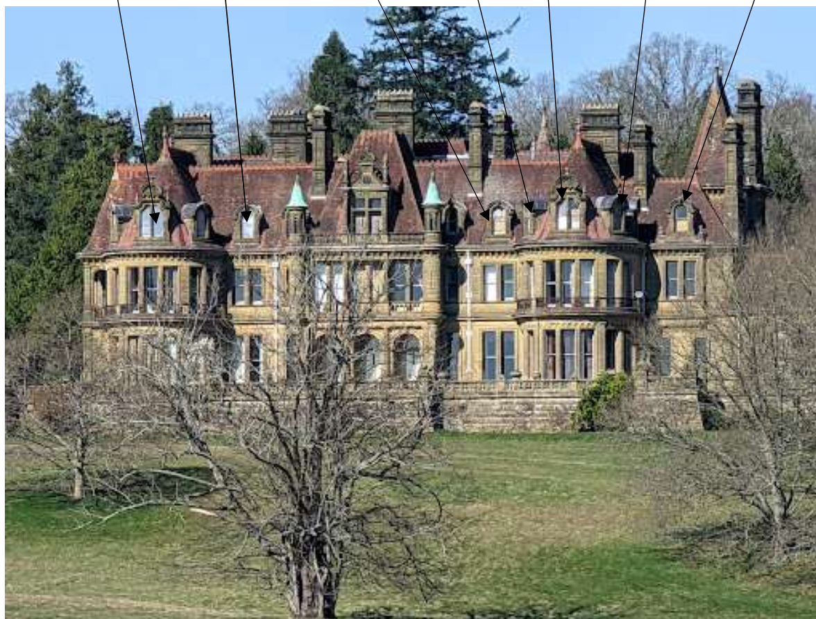
Photo taken from prior to client's acquisition shows the damaged second floor windows generally.
