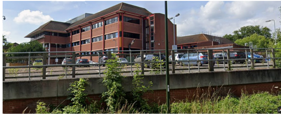
03 External view from Rocky Ln
