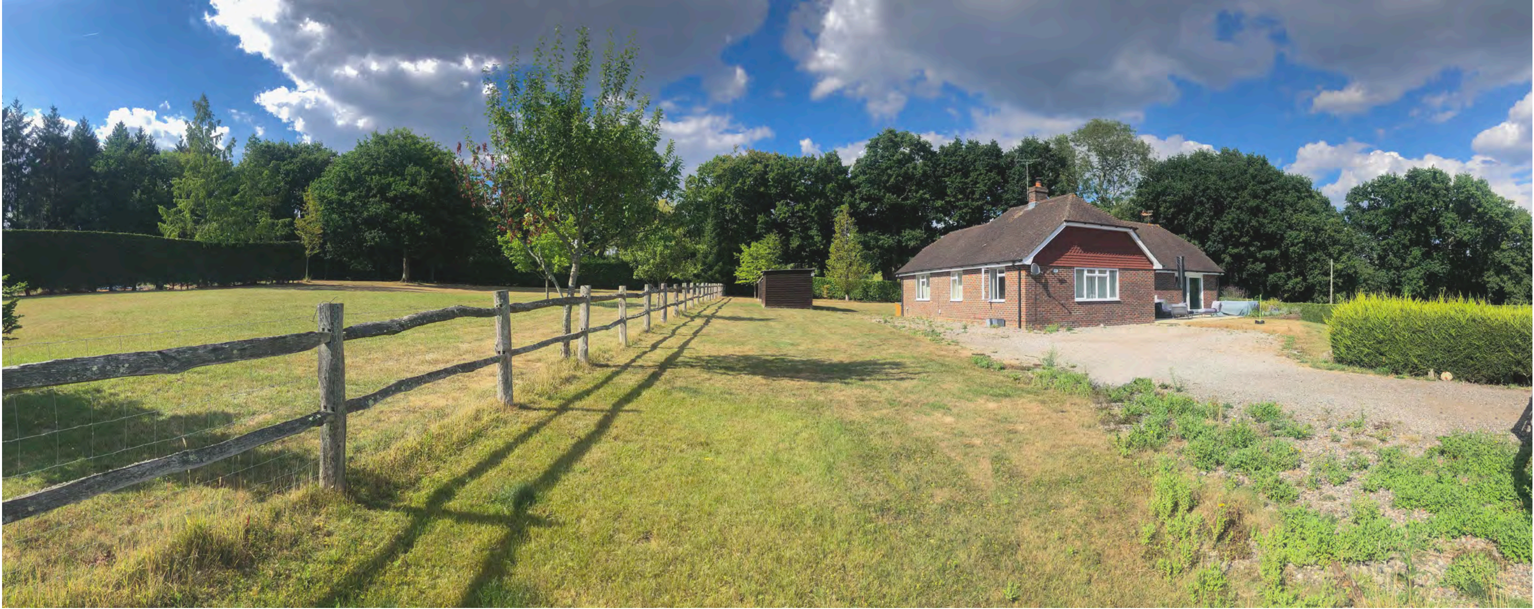
View of existing dwelling looking north east, highlighting its visibility in the landscape and general lack of surrounding vegetation
