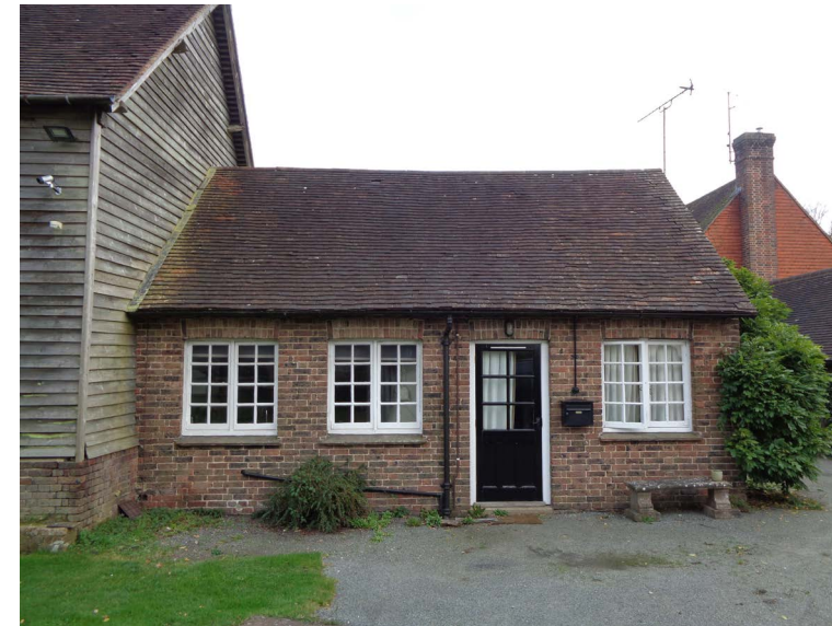
Rear (West Facing) Elevation
