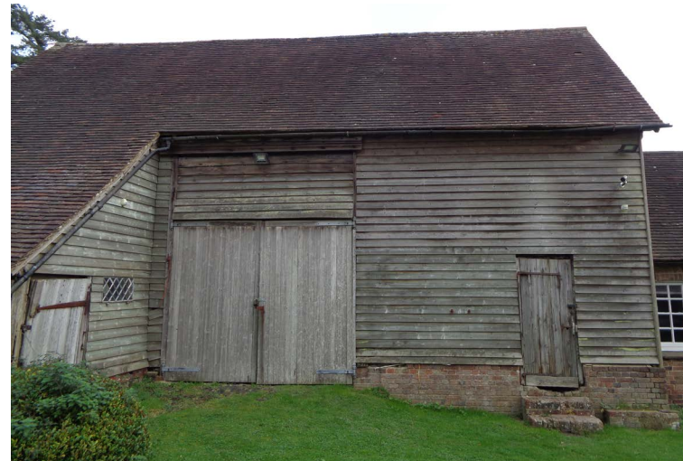
Rear (West Facing) Elevation
