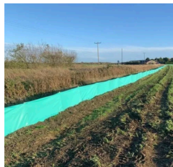
Wildlife friendly “heras” type protective fencing and temporary protective fencing for Newts
