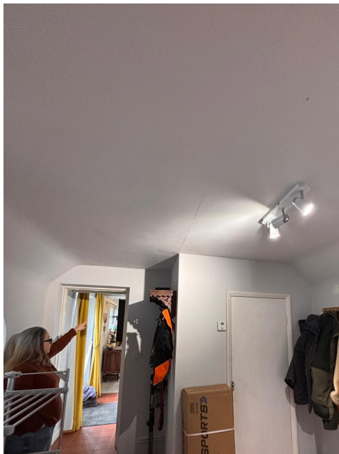
3. Cupboard walls to be removed in bootroom
