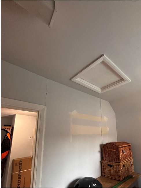
1. Ground Floor Utility Room wall to be removed
