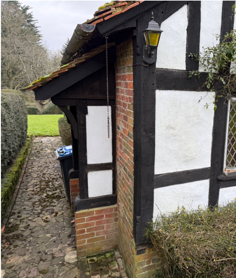
Figure 2 brickwork to C20th range
