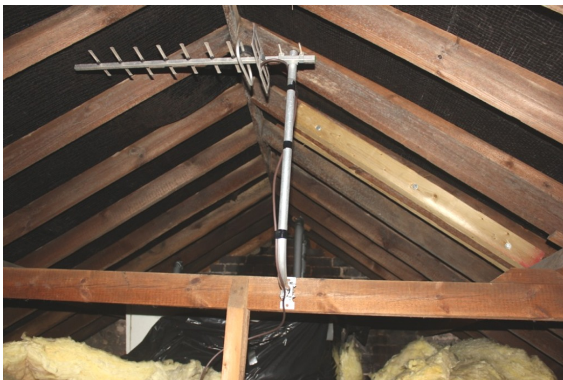
Plate 69. The roof structure, looking north.
