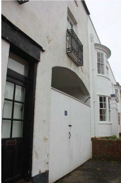
Plate 3. The carriageway entrance looking south-east towards the bow frontage of Lamb House.
