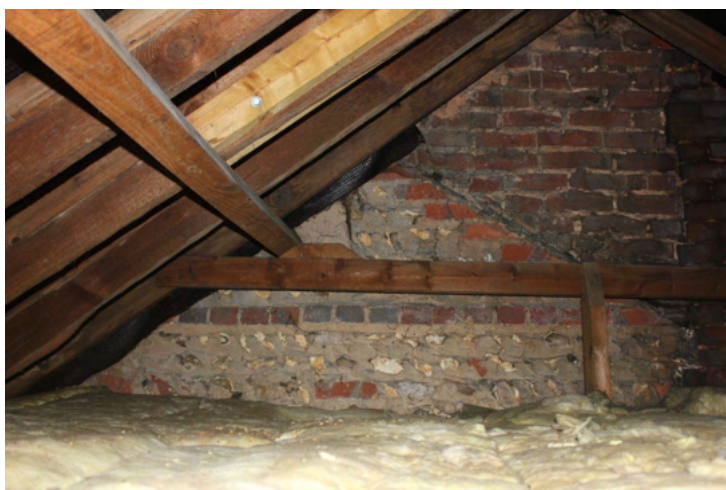
Plate 71. Gable of No. 6 with flint and brick masonry evident as well as the slate roof.
