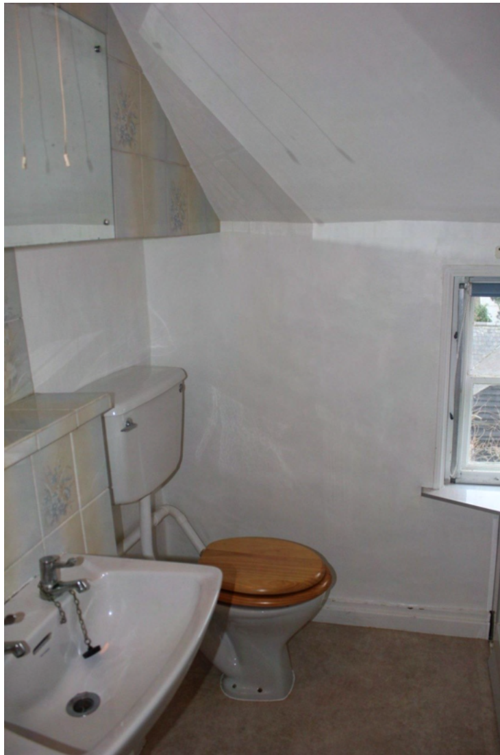
Plate 60. Room S2 with plasterboard wall and skilings.
