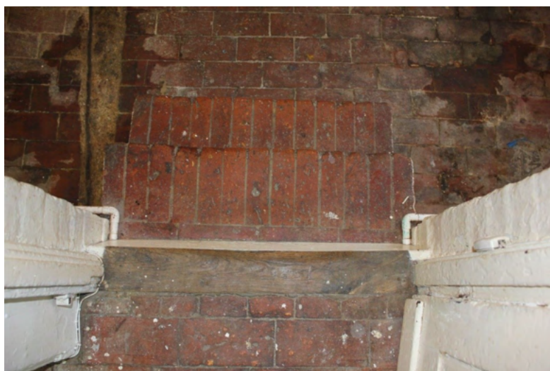
Plate 32. Steps leading down into lean-to with different bricks to the flooring.
