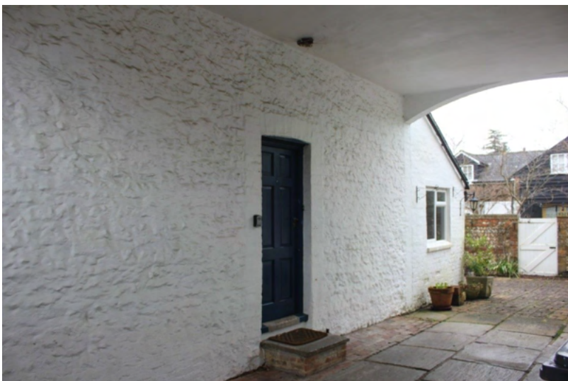
Plate 8. The south facing elevation within the Carriageway.
