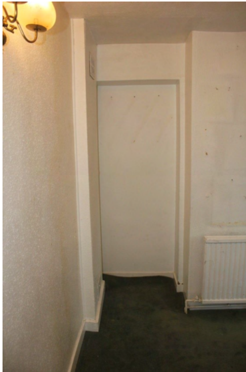
Plate 47. Blocked doorway in the north wall. Plate 48. Partition wall across the stack.
