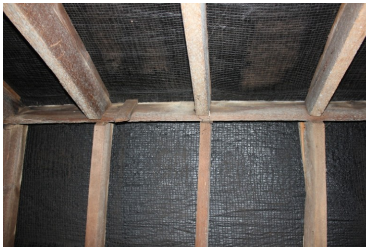
Plate 70. Machined timbers and bitumen lined roof.
