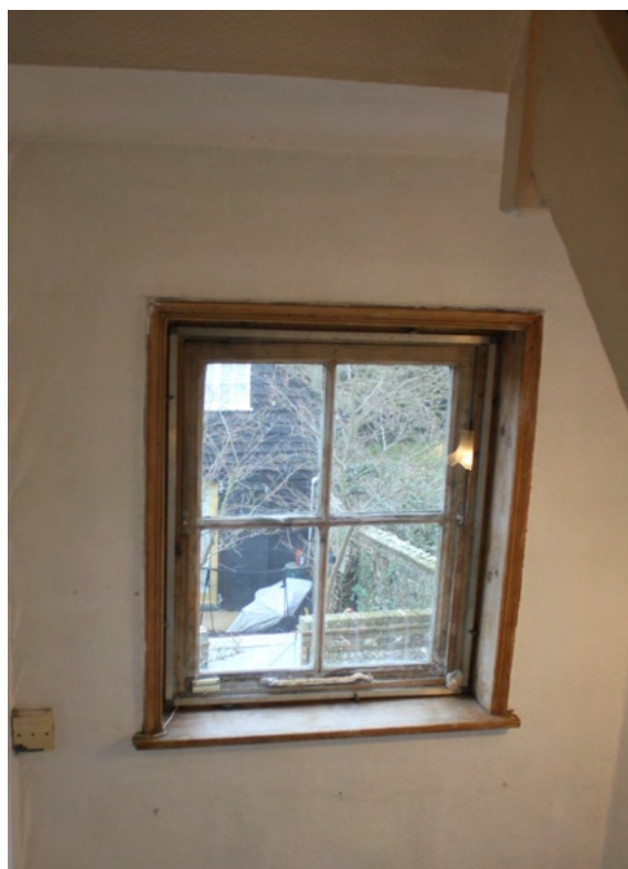
Plate 45. Landing window between ground and first floor levels.
