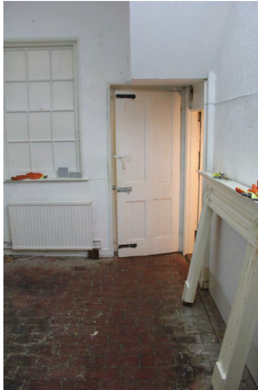
Plate 31. Original brick floor, door into lean-to and painted rear window in Room G2.
