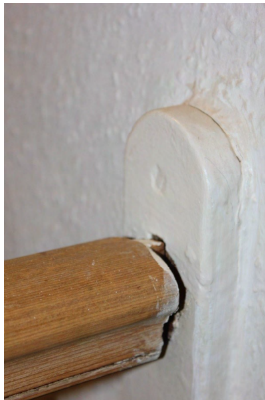
Plate 58. Wall post with rounded top.
