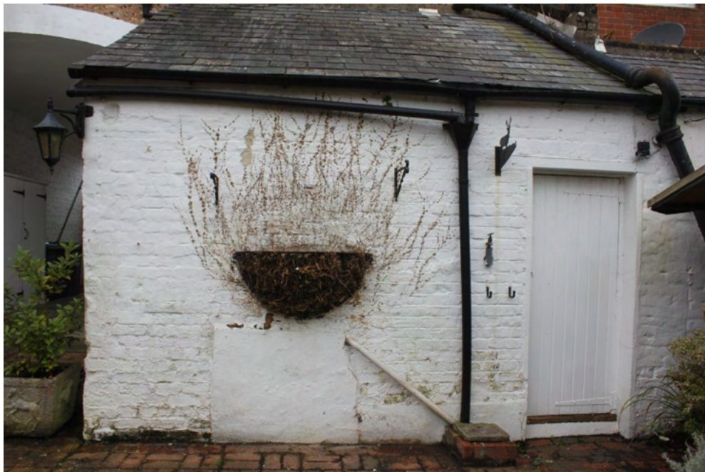
Plate 38. The rear wall of the lean-to.
