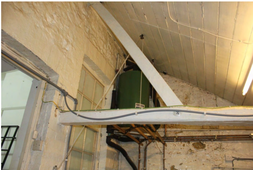
Plate 42. Roof tie and raking strut.
