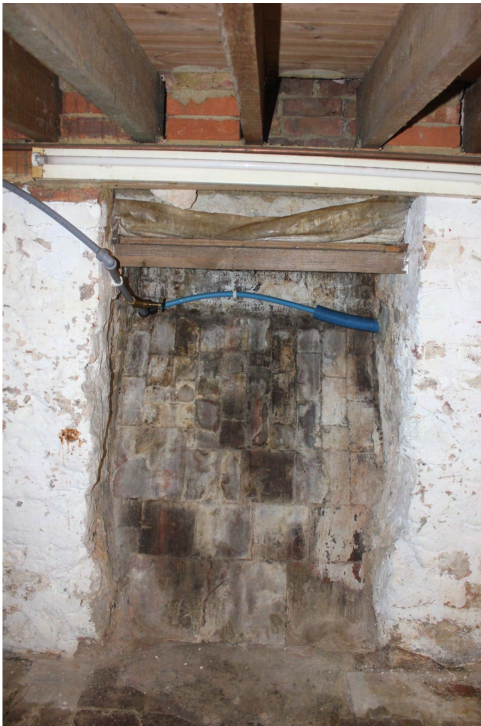
Plate 23. Coal chute in the southern wall.
