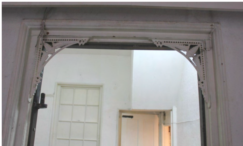
Plate 30. Inserted metal brackets in the doorway.
