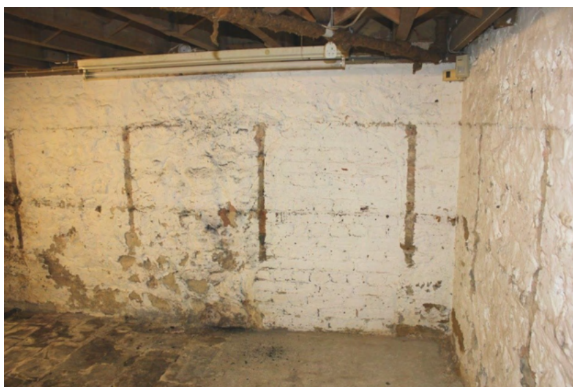
Plate 22. Blocked doorway in the north wall, adjacent to the hearth above.
