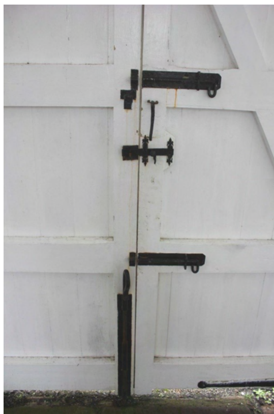
Plate 18. The rear of the Carriageway doors.
