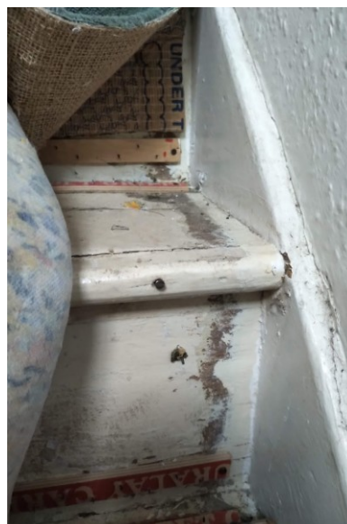
Plate 37. 20 th century, bull-nosed stair treads.
