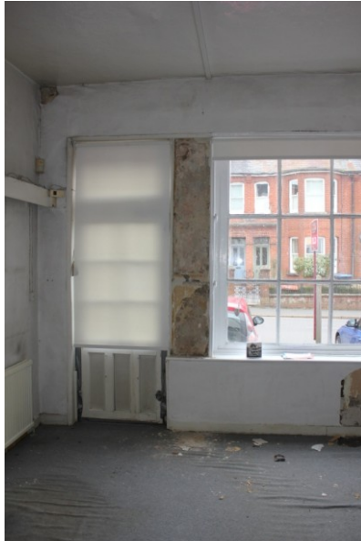
Plate 25. The replacement door and window to the front.
