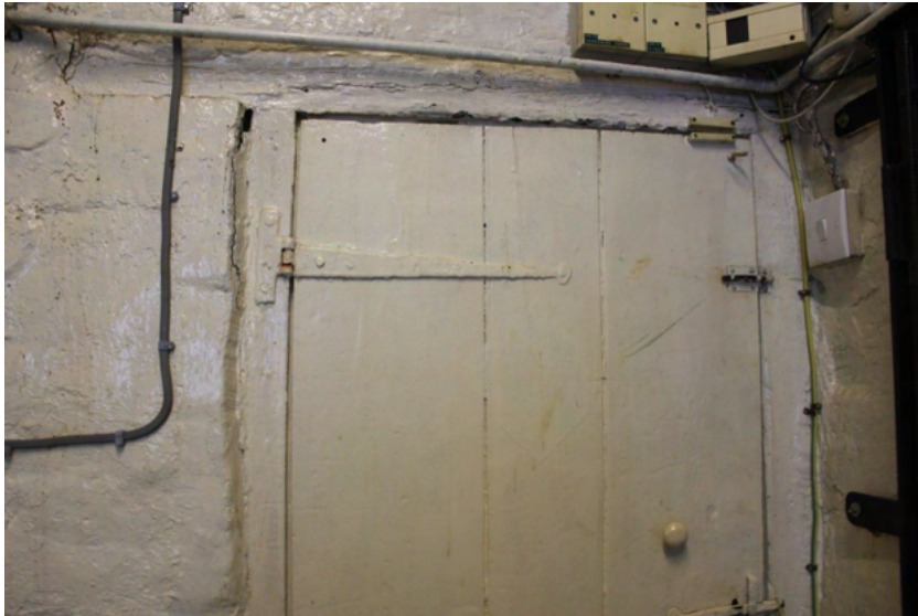
Plate 41. Door leading into the toilet.
