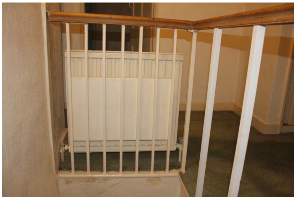
Plate 56. Surviving in-situ balusters and slender newel post.
