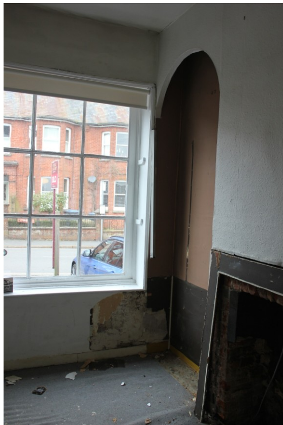
Plate 28. Modern arches built into the alcoves.
