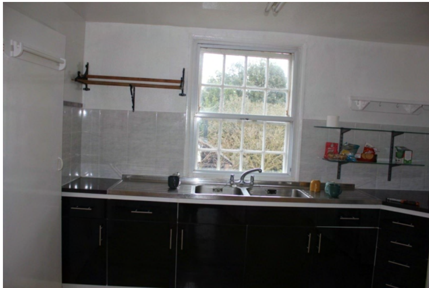
Plate 53. Original six over six sliding sash window in the east wall of Room F5.
