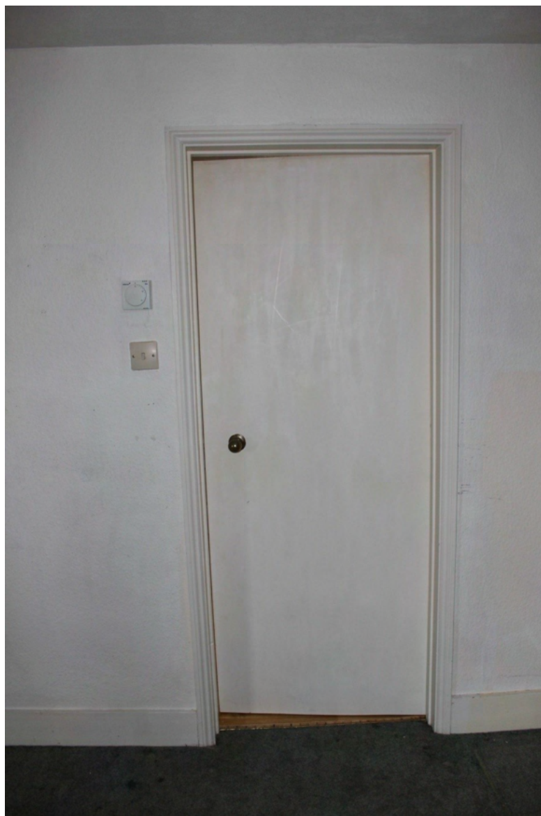
Plate 52. Original architrave but modern door in the doorway leading into Room F5.
