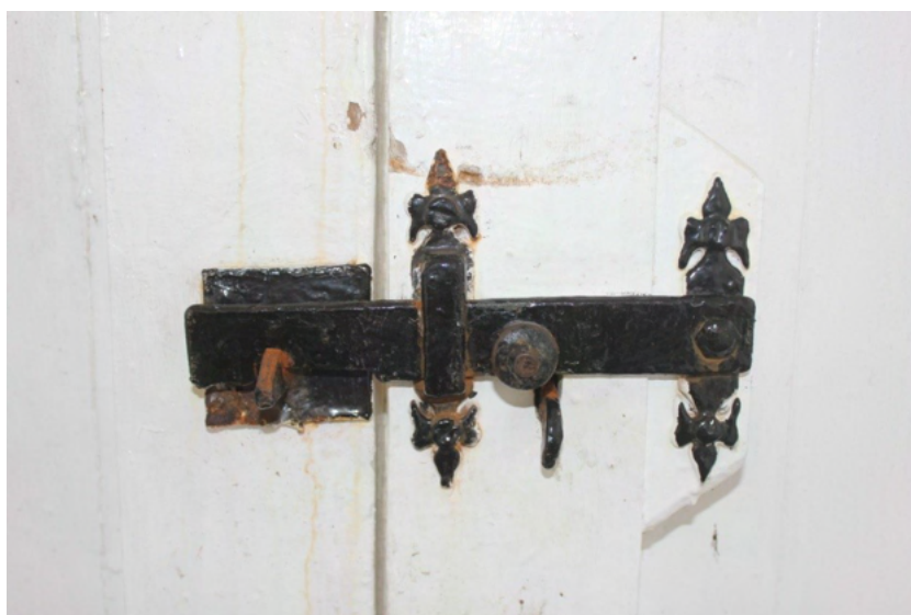
Plate 19. Replacement door latch.
