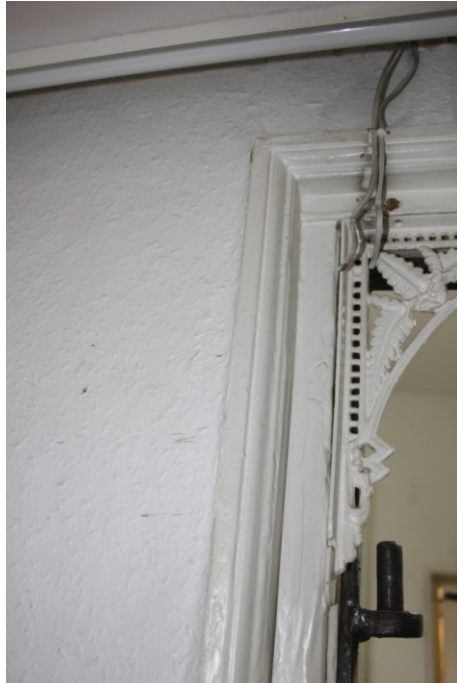
Plate 29. Original architrave in the doorway between Room G1 and G2.
