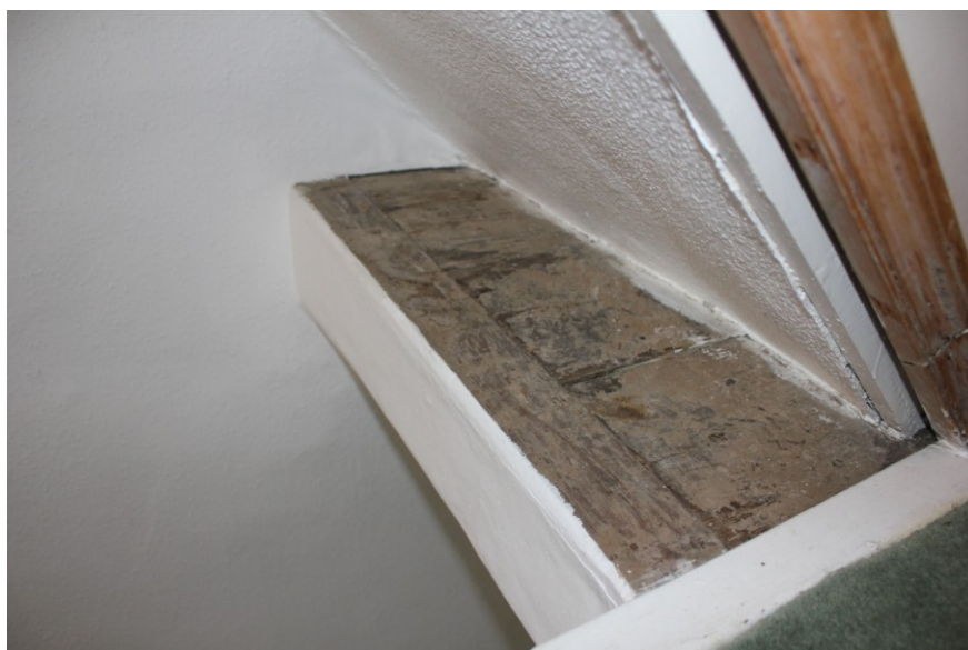
Plate 46. Small section of original floorboards within the first floor landing.
