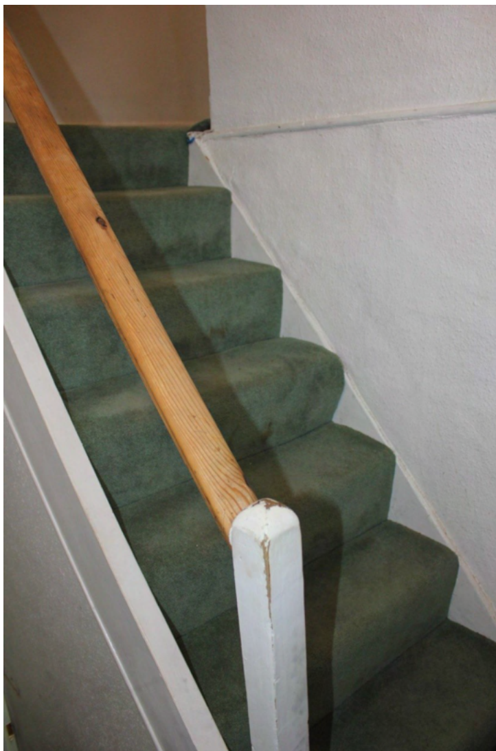
Plate 44. 20 th century newel post and stairs with re-used handrail.
