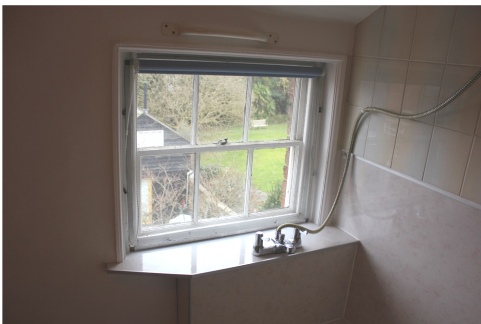
Plate 61. Original sliding sash window in the east wall.
