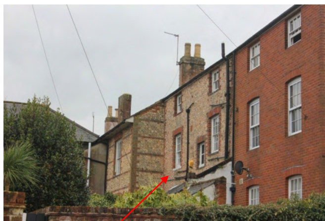
Plate 4. The rear, east facing elevation of the Coach House in flint with brick dressings.
