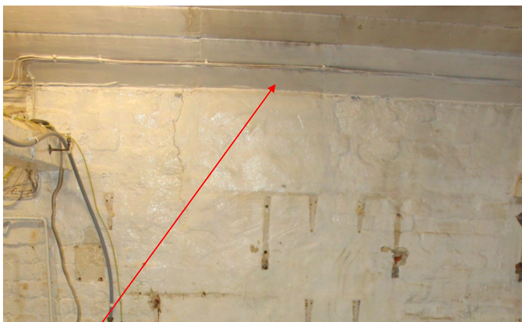
Plate 40. Patch in roof for removed stack and rendered wall showing former stack outline.
