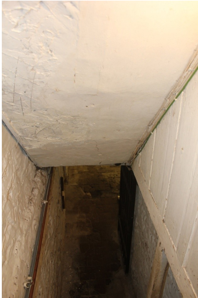
Plate 24. Underside of the stairs leading to the first floor.
