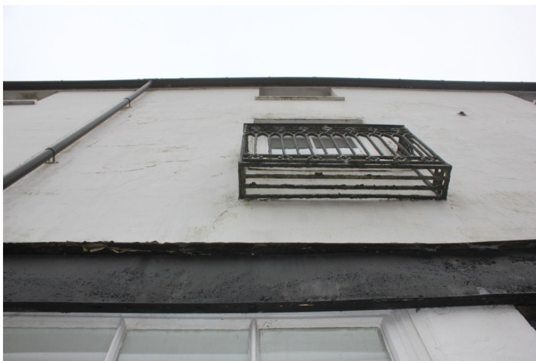
Plate 13. Looking up underneath the balconies.
