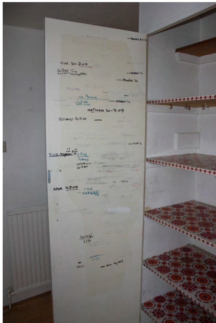
Plate 54. Cupboard in the north wall of Room F5 with lath and plaster to the rear.
