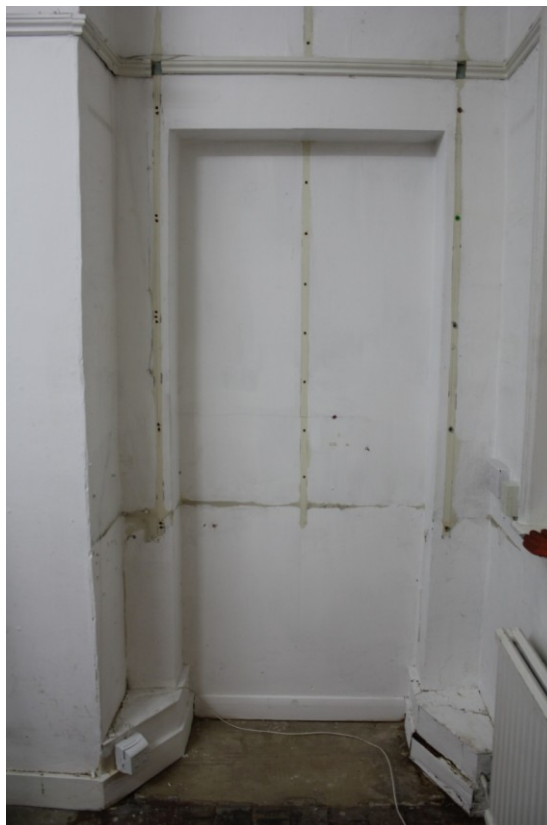
Plate 33. Blocked doorway in north wall of Room G2.
