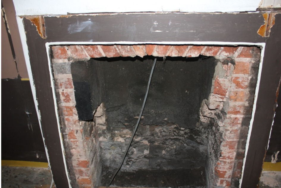
Plate 27. Possible original fire fascia with alterations to the aperture.
