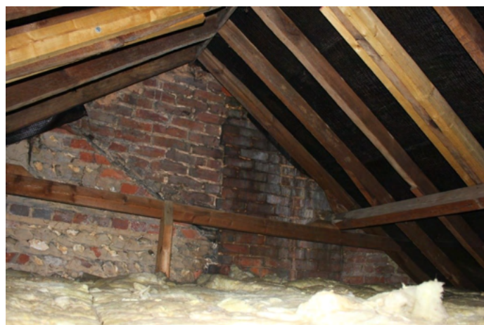
Plate 72. Infill brickwork in the southern gable.
