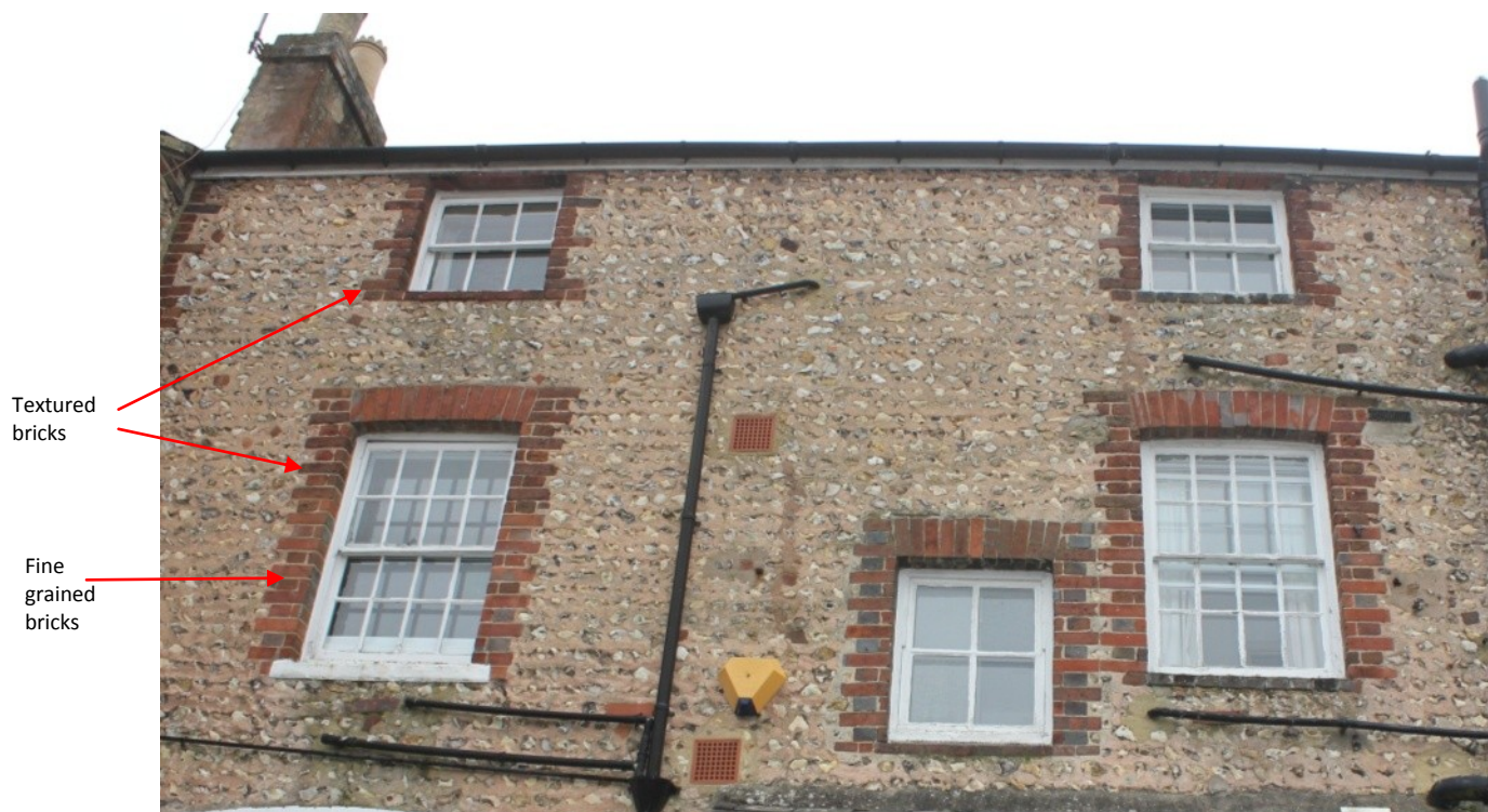
Plate 14. Brick dressings with two brick types present.
