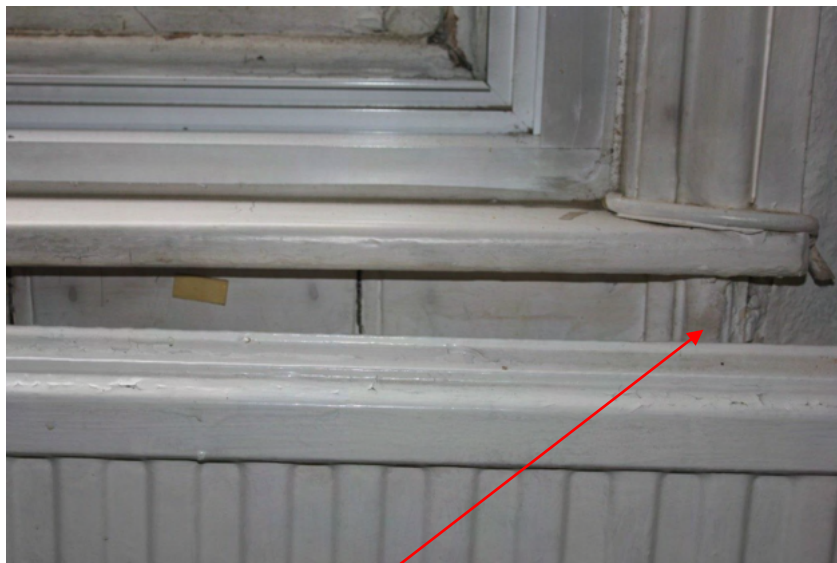
Plate 50. Different architrave and boarding glimpsed below the window.
