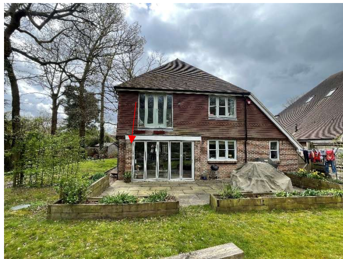
Image of the rear façade and location of single-story extension
