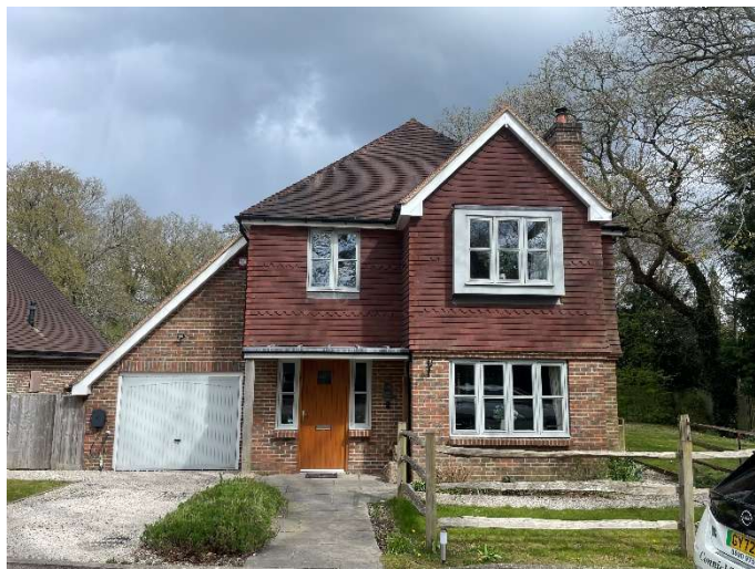
Image of the front façade
