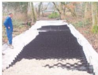
CellWeb during installation.
