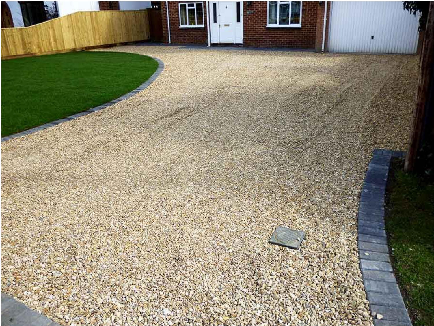
Buff Colour Shingle to external area where rear extension is to be removed
