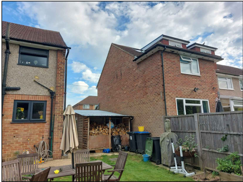
4 - Rear elevation looking to No. 77
