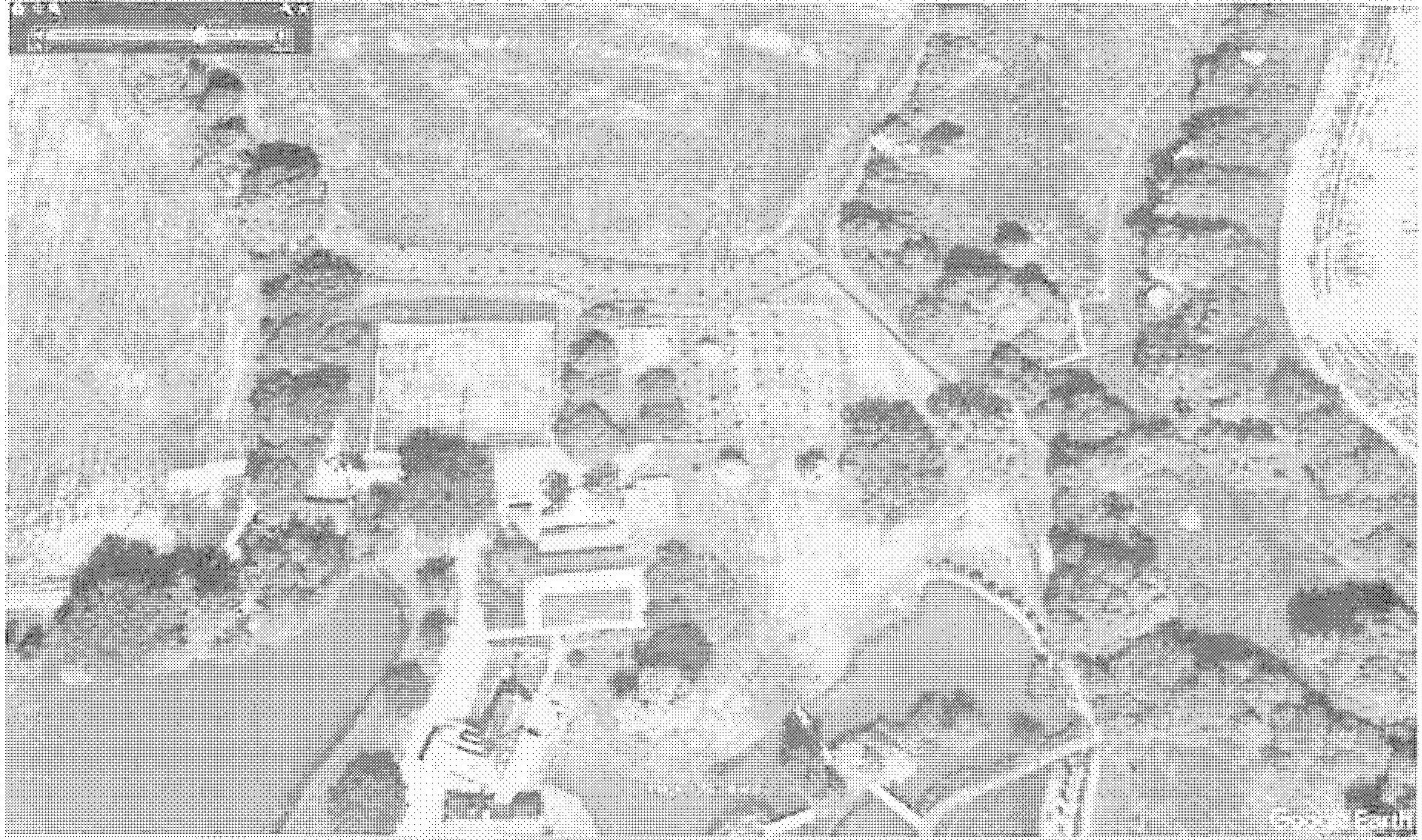
Photo Above: Dated September 2012 shows the 4 Bay Garage, Double Garage & Outbuilding in situ.
