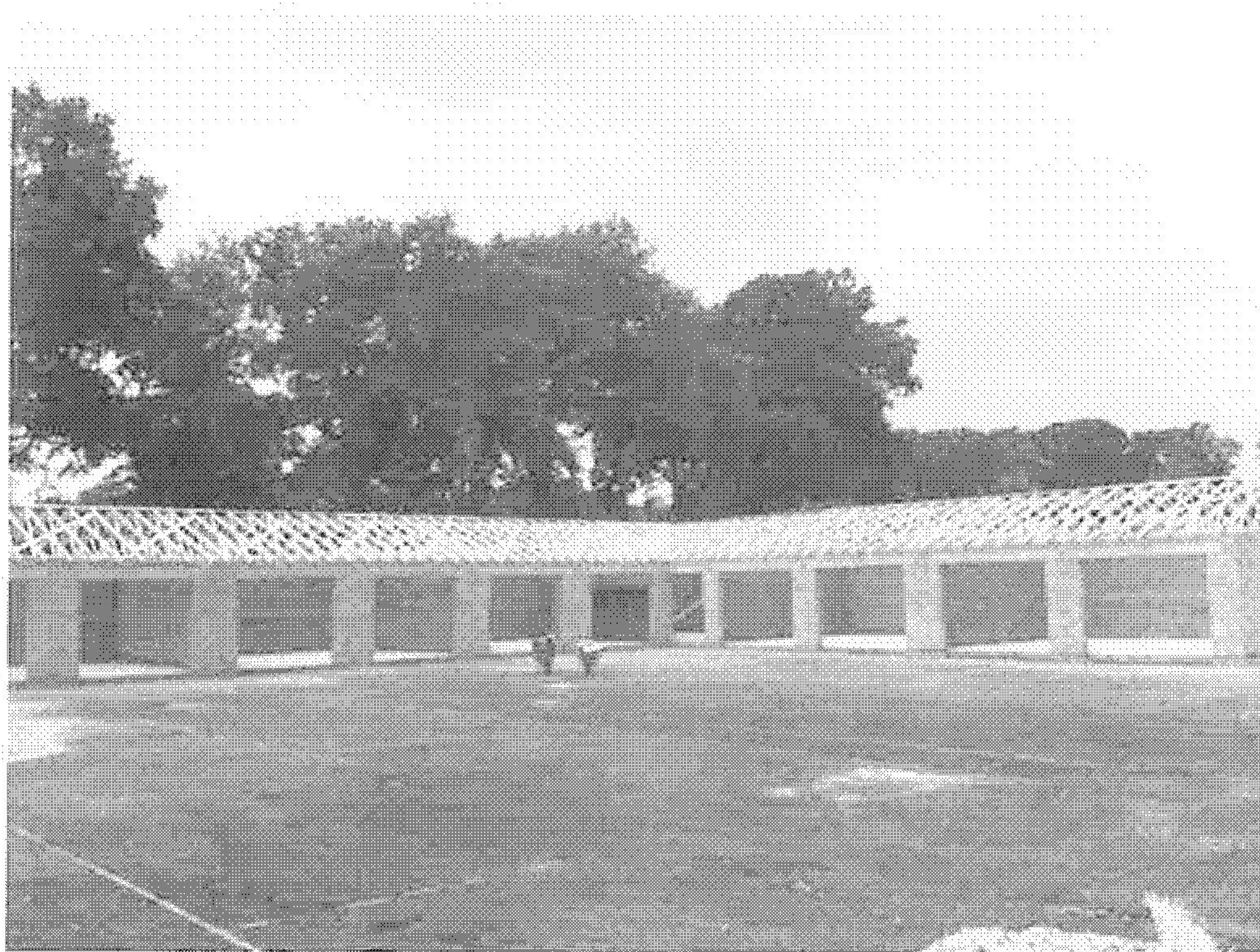
Photo Above: Dated 8 th August 2014 showing the walls and roof structure of the main garage block erected.
