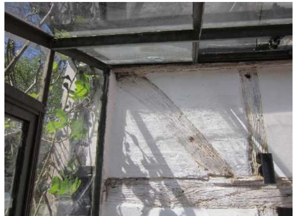
Figure 5; external view of the square panel framing of the east wall of the first floor chamber, bay 3, showing (from top to bottom) a midrail, a down brace, a stud, and a girt.
