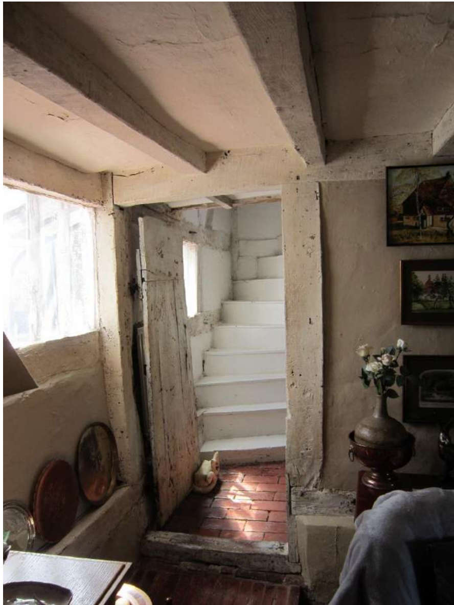
Figure 15; the doorway from the hall into the service bay, and also showing the stairs to the chambers over. The two rare surviving open mullioned windows are also visible on the left-hand side. The nearest one providing light into the hall and the furthest one providing light into the service room.
