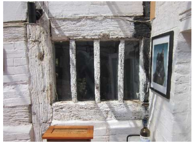
Figure 17; external view of the hall window. 810mm wide by 580mm with nominal centres of 220mm
