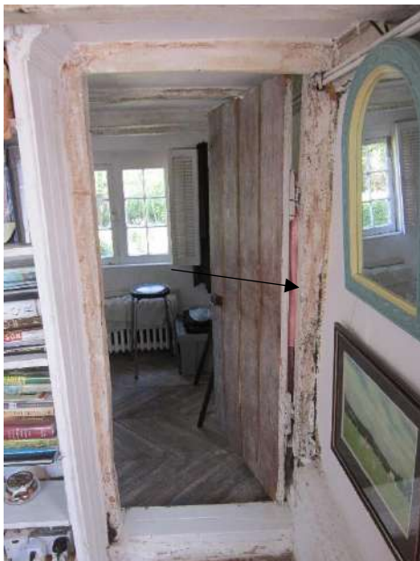
Figure 31; door hung on an elm stud, against the back of the cross-frame between bays 2 and 3.
