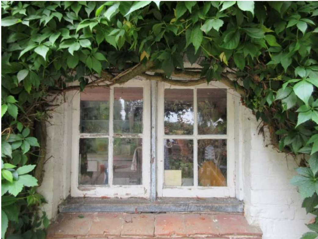
Figure 14: Rear (east) elevation – kitchen window.
