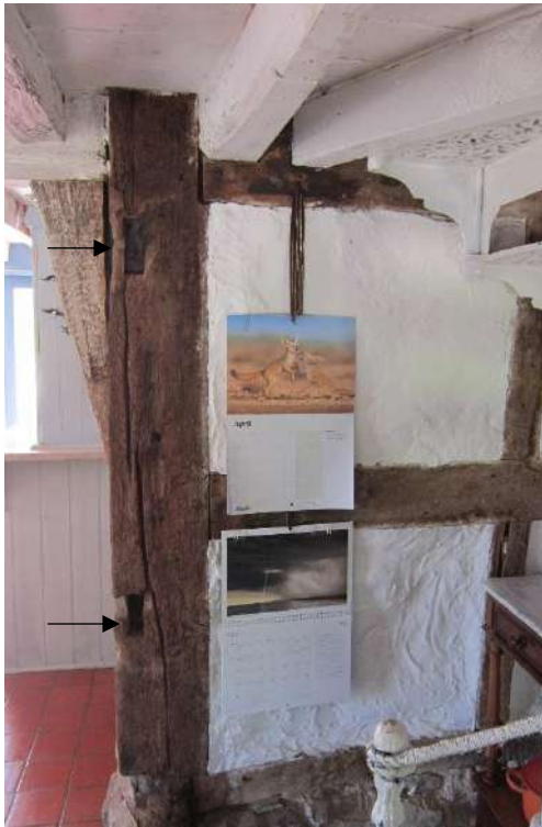
Figure 20; the north-east bay post, with its two empty mortices and square panel framing of the cross-frame between the smoke bay and the lean-to.
