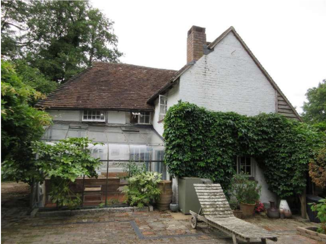
Figure 12: Rear (east) elevation of house.
