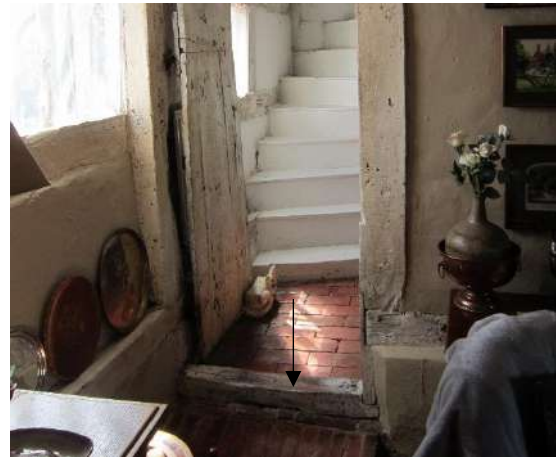
Figure 36; showing the step between the lower floor of the hall and higher floor of the service room.
