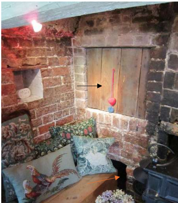
Figure 24; showing the opening for the former bread oven above and niche for the ashes below.
