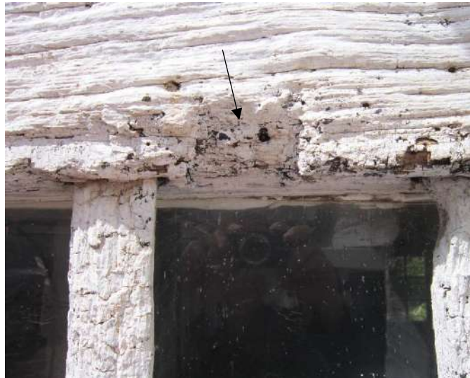
Figure 34; notch formed when a stud was inserted on the external face of the framework and probably lathed over to enclose the hall window.
