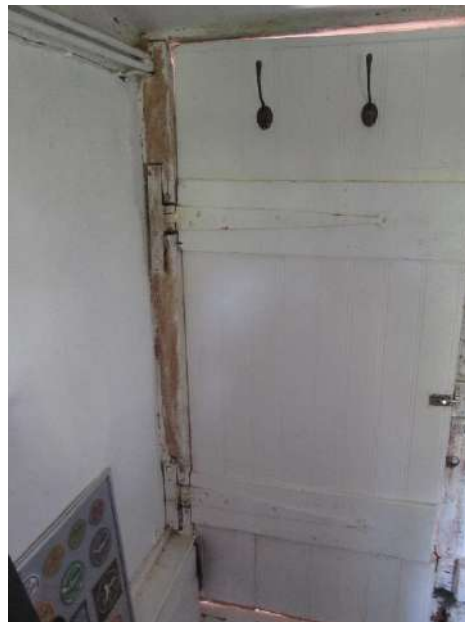
Figure 32; the cross-garnet or T hinges used to hand the new door on.
