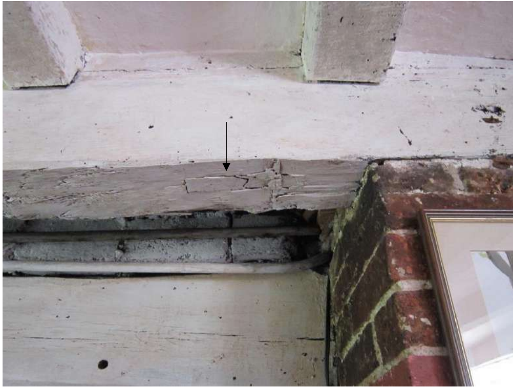
Figure 8; the sawn off tenon for the stud that formed the dividing wall between the framed chimney and the baffle entrance. This framed chimney had an internal width of about 2.2m (7'6").
