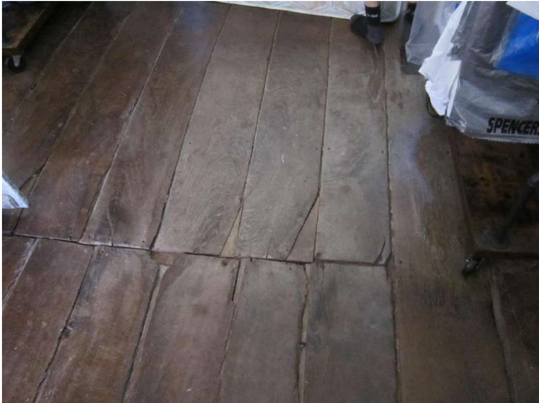
Figure 14; the oak floorboards over the hall are likely to be original, based on their species, size, arrangement and nail pattern.
