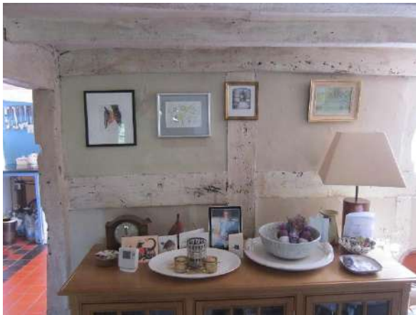
Figure 4; internal view of the square panel framing of the east wall of the ground floor hall, bay 2, showing vertical studs and midrails.
