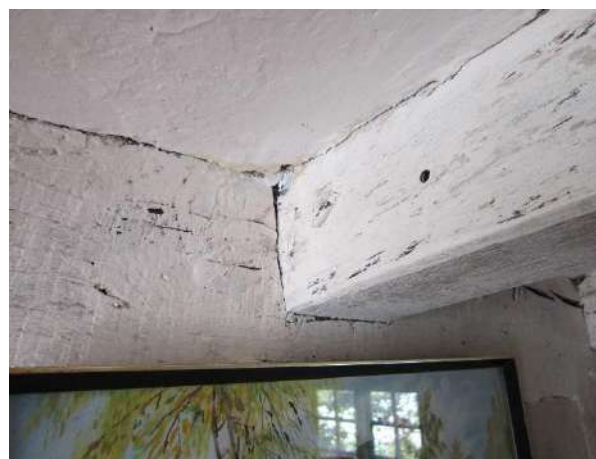
Figure 13; The tenoned end of a hall floor joist where it joints into the transverse beam of cross-frame 3, at the high end of the hall.
