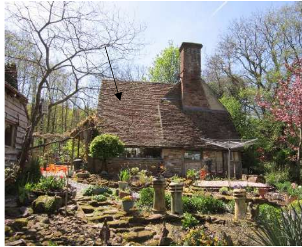
Figure 30; the range built against the east wall and abutting the Phase B lean-to. Note the shallower roof slope of this range compared to the earlier phase.
