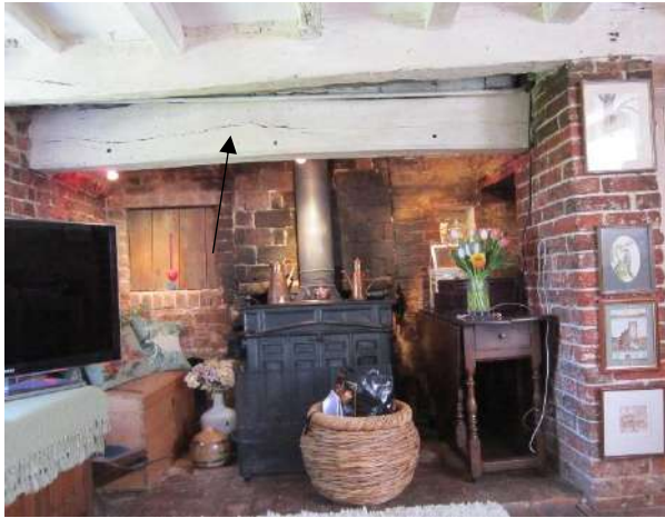
Figure 22; new oak mantlebeam (from a reused timber) with brick chimney.
