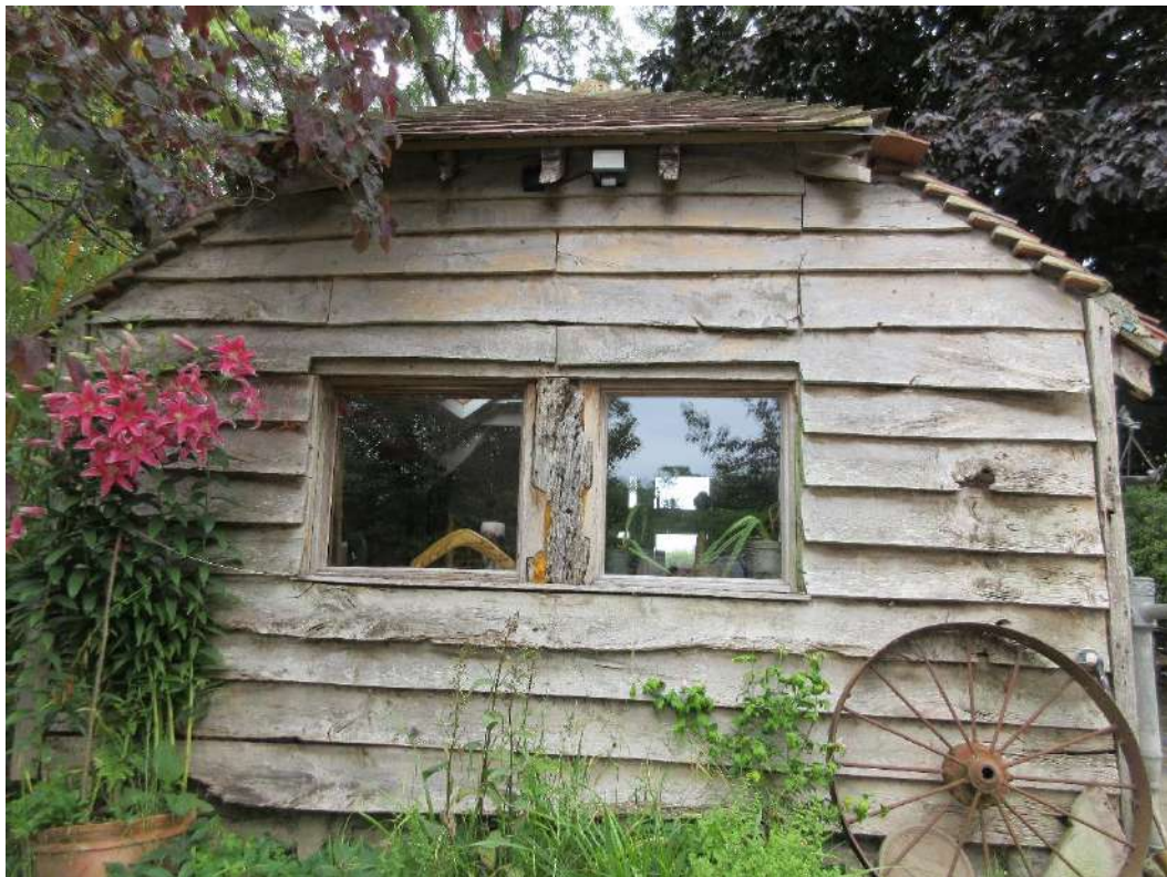
Figure 61: Side (west) elevation of annexe.
