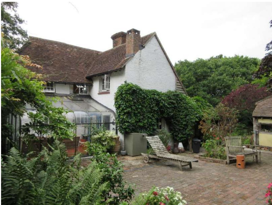
Figure 18: North-westward view of rear terrace, with rear (east) elevation of house.
