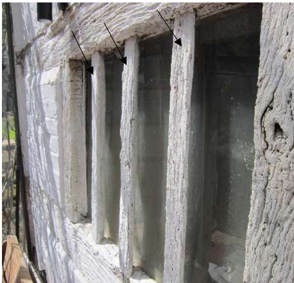
Figure 18; showing the triangular cross-section of the three service room mullions.
