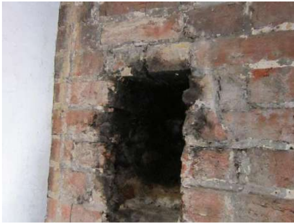
Figure 26; possible entry of a flue for a copper into the main chimney.
