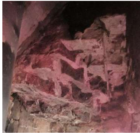
Figure 27; possible flue for a copper within the main chimney. Some bricks have been removed and some hacked back, at a later date.
