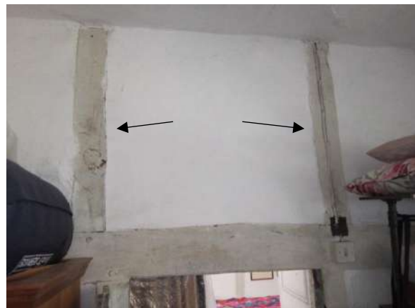
Figure 3; the two queen struts on the cross-frame between bays 2 and 3.
