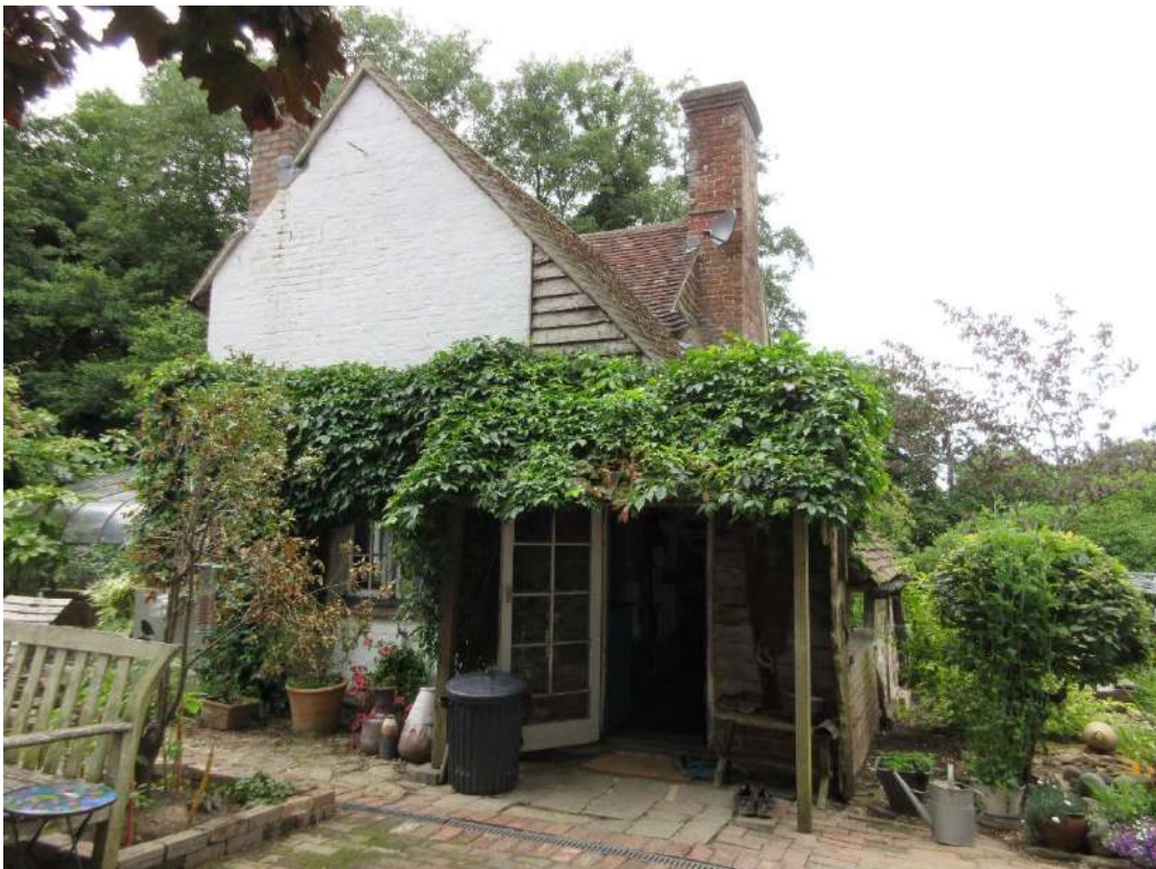
Figure 13: Rear (east) elevation of house (i.e. 19 th century extension).
