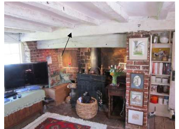
Figure 7; the transverse beam of the framed chimney (arrowed) forming the front of the smoke bay in the hall.
