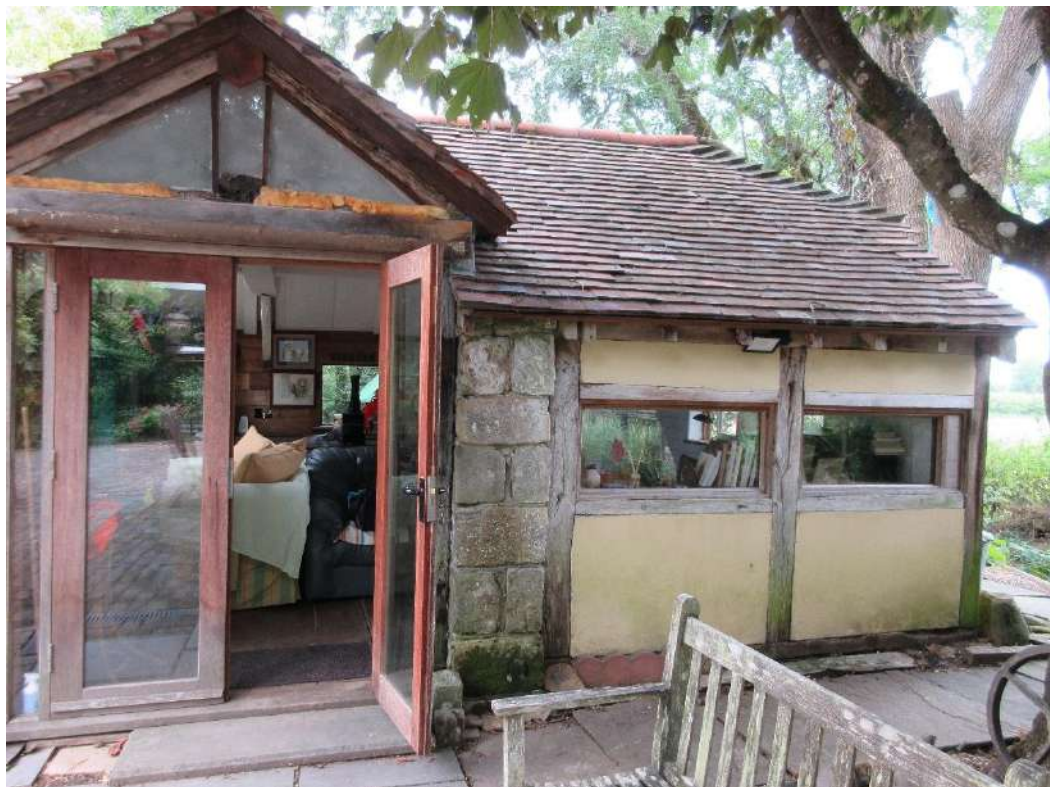
Figure 58: Front (south) elevation of annexe.
