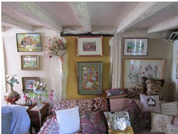
Figure 6; the cross-frame at the high end of the hall, showing only vertical studs, 3 number, and no midrails.
