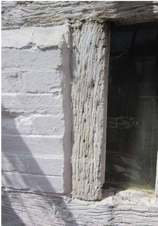
Figure 33; nail evidence, probably for laths, on a stud of the service window.
