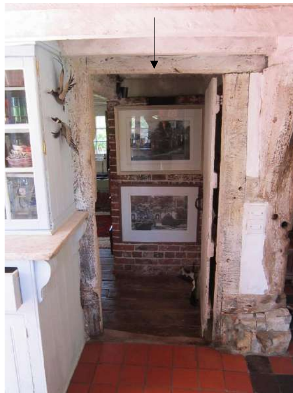
Figure 9; the location of the original front doorway into the house, forming a baffle entrance that leads into the floored hall.
