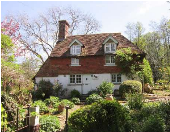
Figure 35; showing the weather-tiling and dormers on the west elevation.
