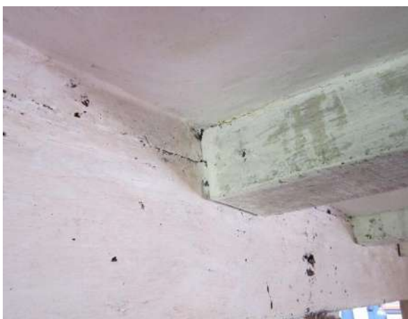
Figure 12; the notched end of a hall floor joist where it lodges over the transverse beam of the framed chimney. This allows the joists to be inserted once the main structural frame has been reared up.
