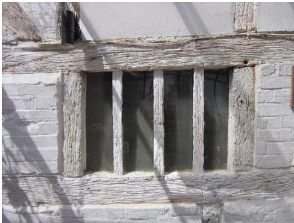
Figure 16; external view of the service room window. 825mm by 580mm with nominal centres of 220mm
