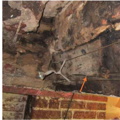
Figure 23; internal view of the mantlebeam showing the typical large chamfer associated with these timbers.
