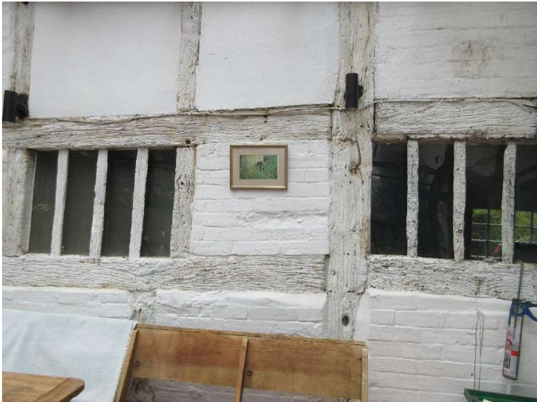
Figure 40: House interior – Conservatory, with original external wall and windows (with original mid to late 16 th century timber mullions).
