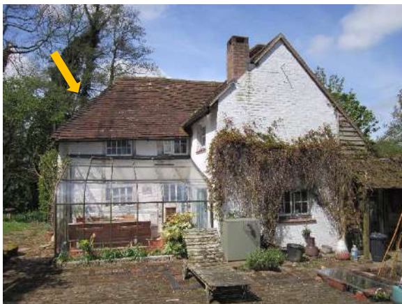
Figure 2; the hipped terminal of the south end of the cottage.
