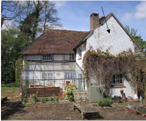
Figure 29; the range built against the east wall, viewed from the east.
