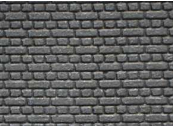
Black Painted Brickwork English Bond
