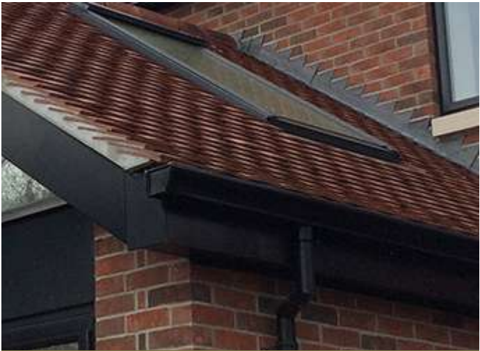
Black Timber Fascia
