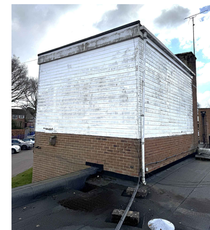
VIEW 1 - North-West View on Tank Room (N.T.S.)
