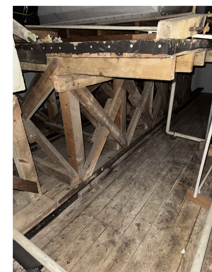
VIEW 6 - 1st Floor view from south-east corner (N.T.S.)
