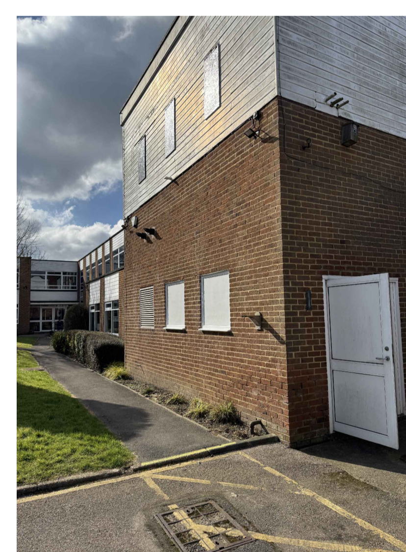
VIEW 4 - North-East View 2 on Tank Room (N.T.S.)
