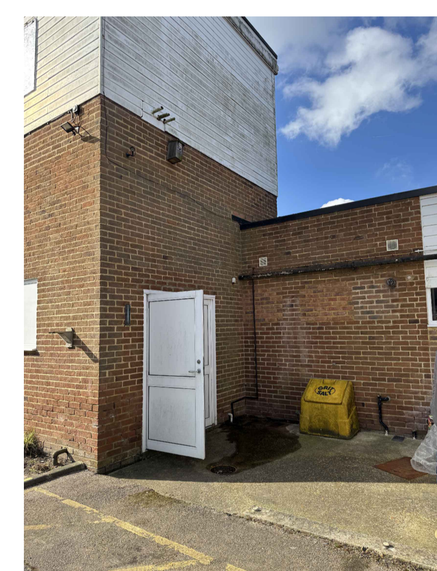
VIEW 3 - North-East View 1 on Tank Room (N.T.S.)
