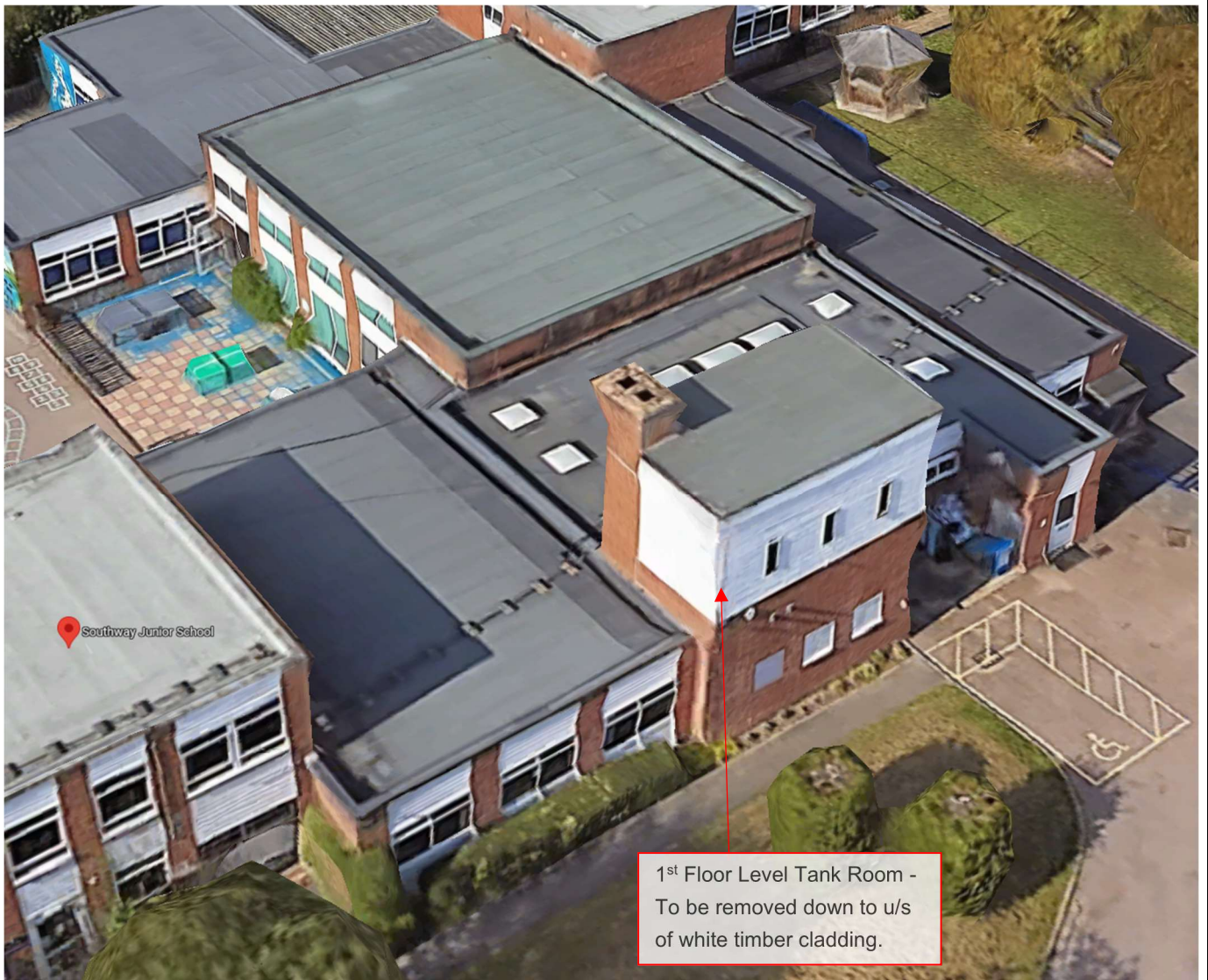
Fig. 1 – South East Aerial View on Southway Junior School – Showing 1 st Floor Level Tank Room
