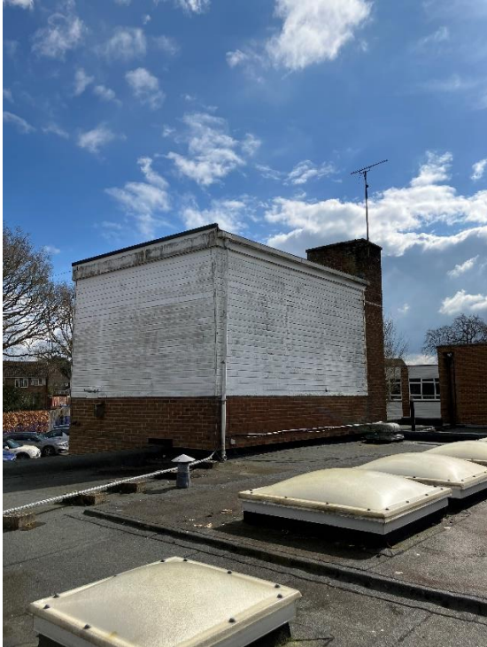
Photo 1: North and East Facing Elevation
