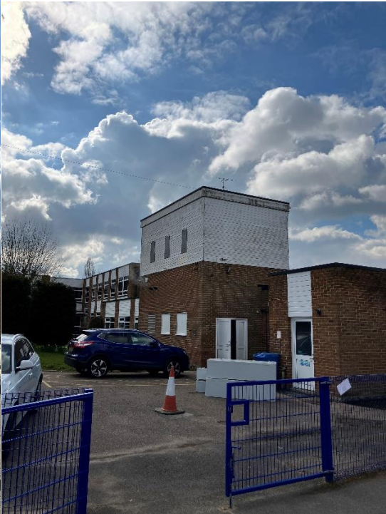
Photo 2: North and West Facing Elevation
