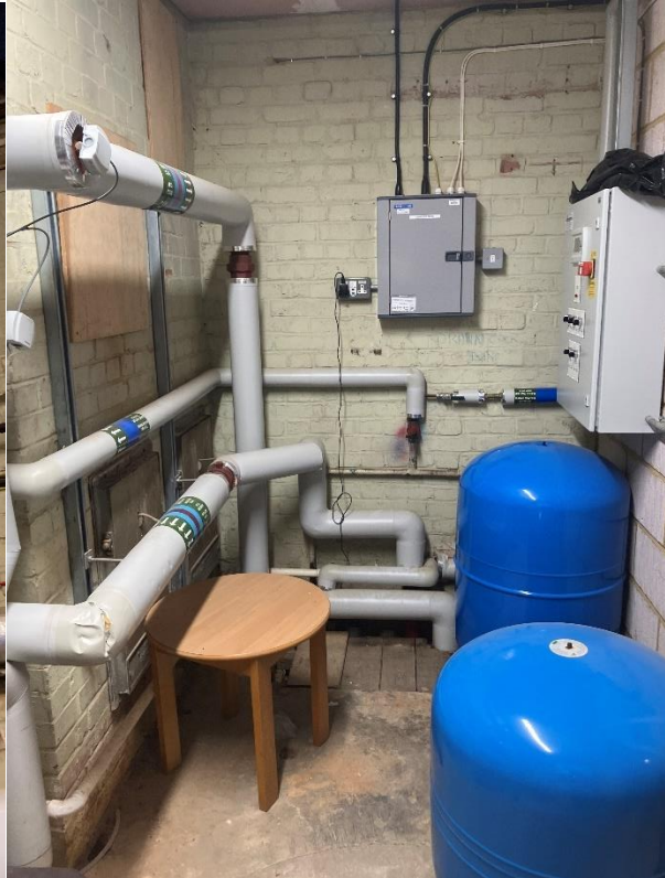
Photo 10: Internals 075 plant room and redundant chimney stack
