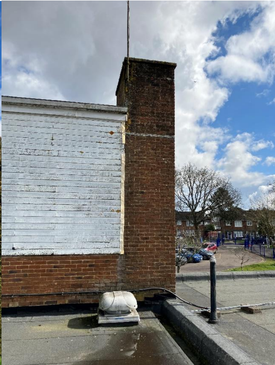
Photo 4: West Facing Elevation
