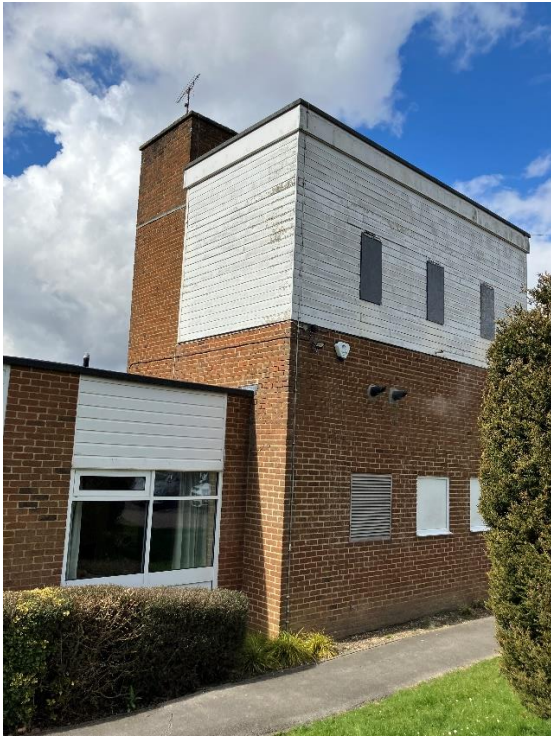
Photo 3: South and West Facing Elevation
