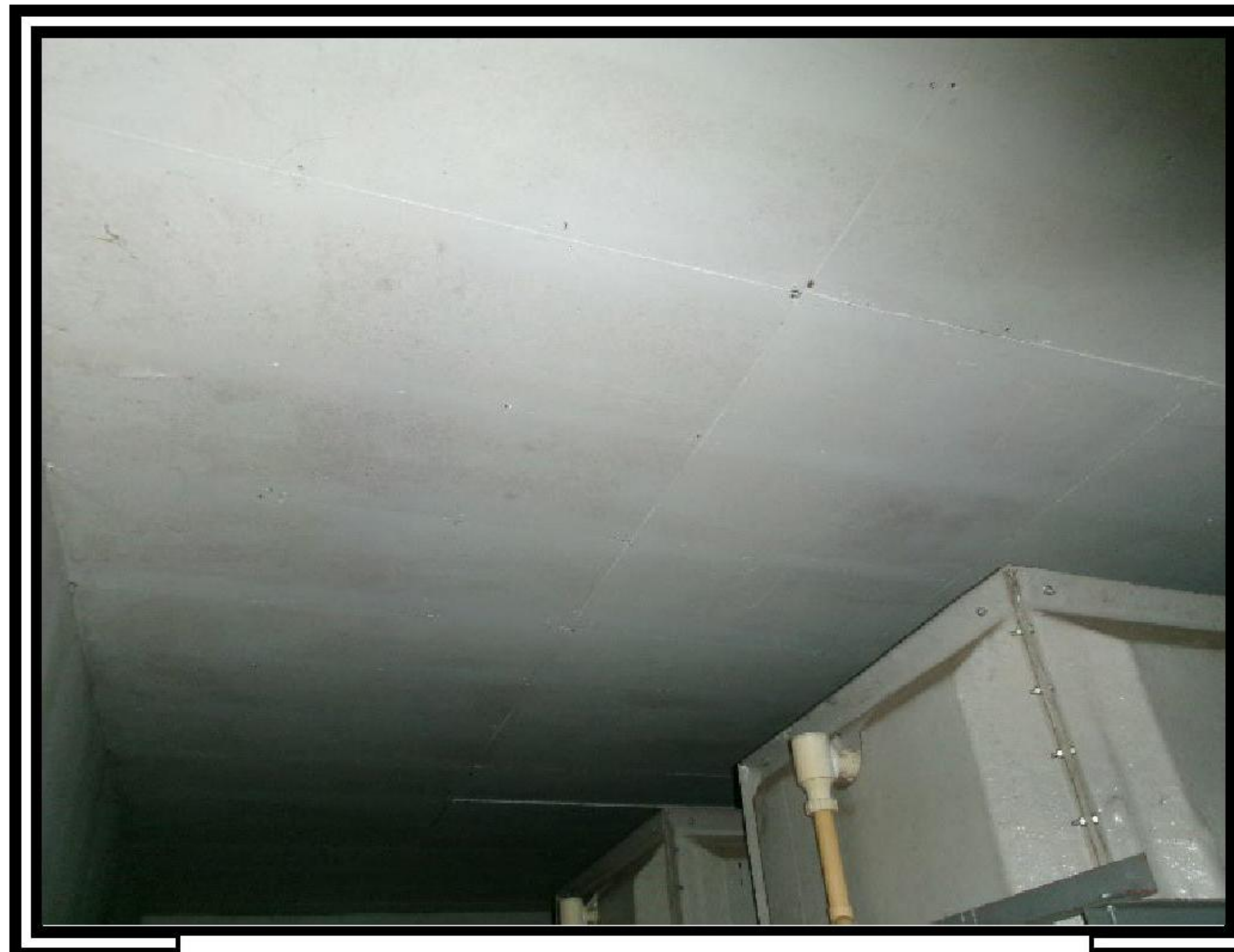
Asbestos insulating board ceiling panels
