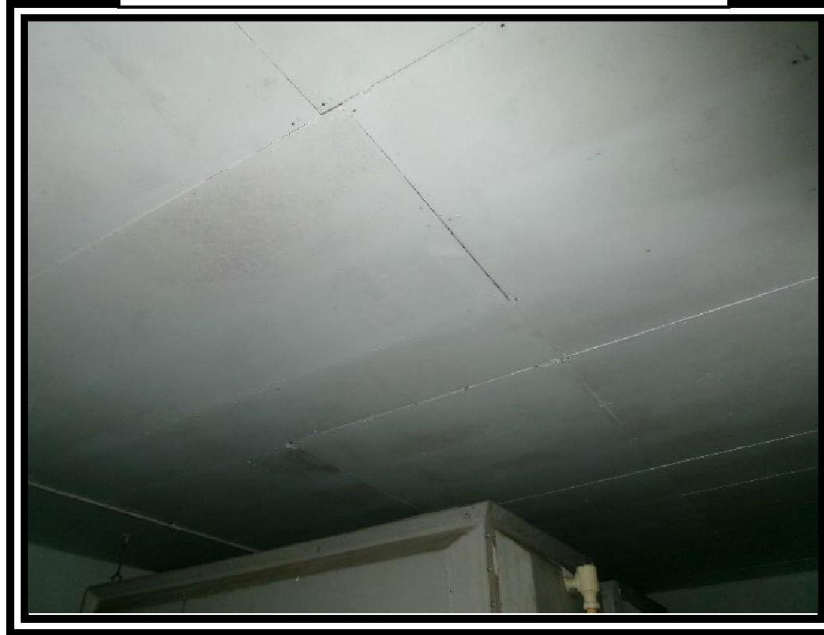
Asbestos insulating board ceiling panels
