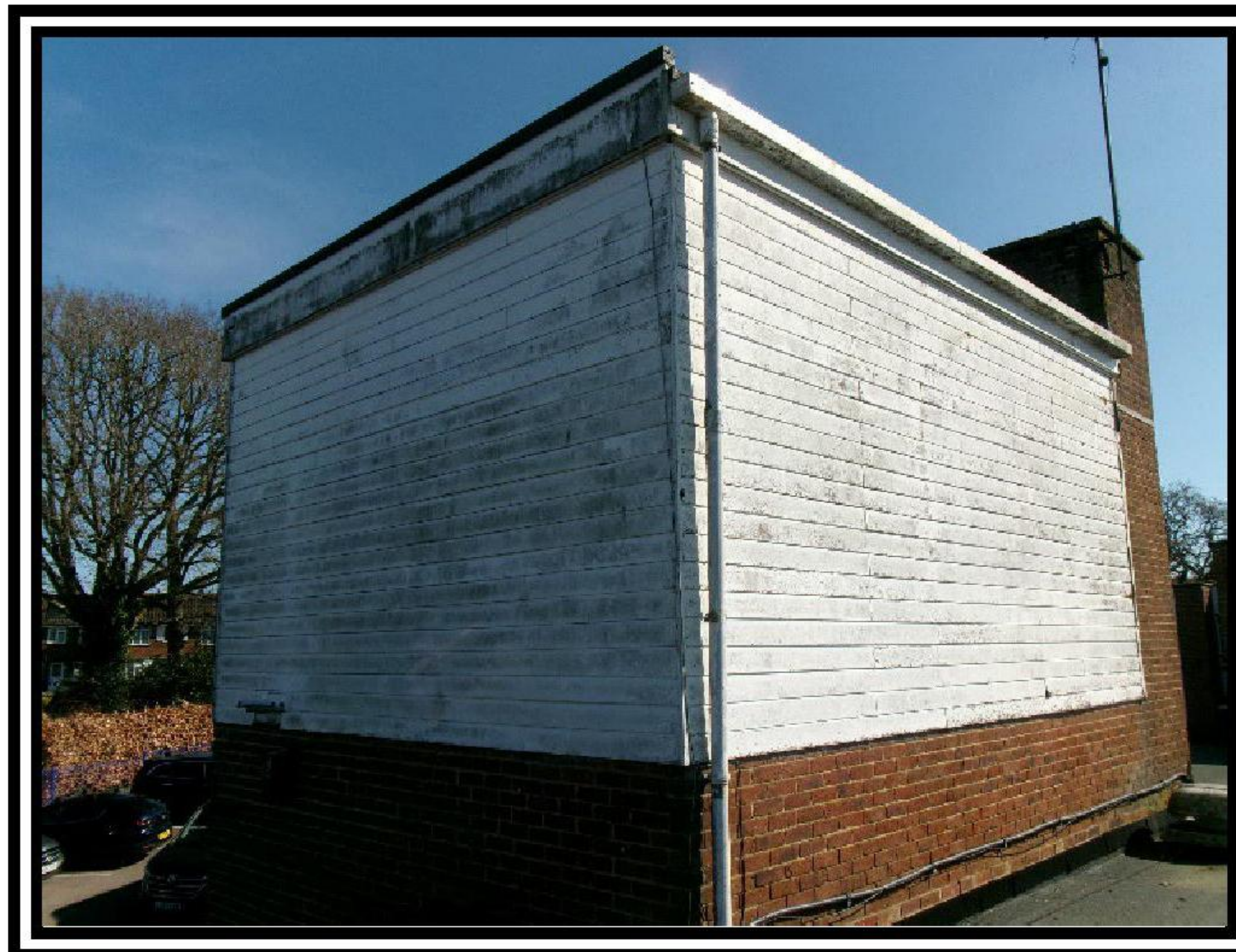
Asbestos cement shiplap panels to 072 Tank Room
