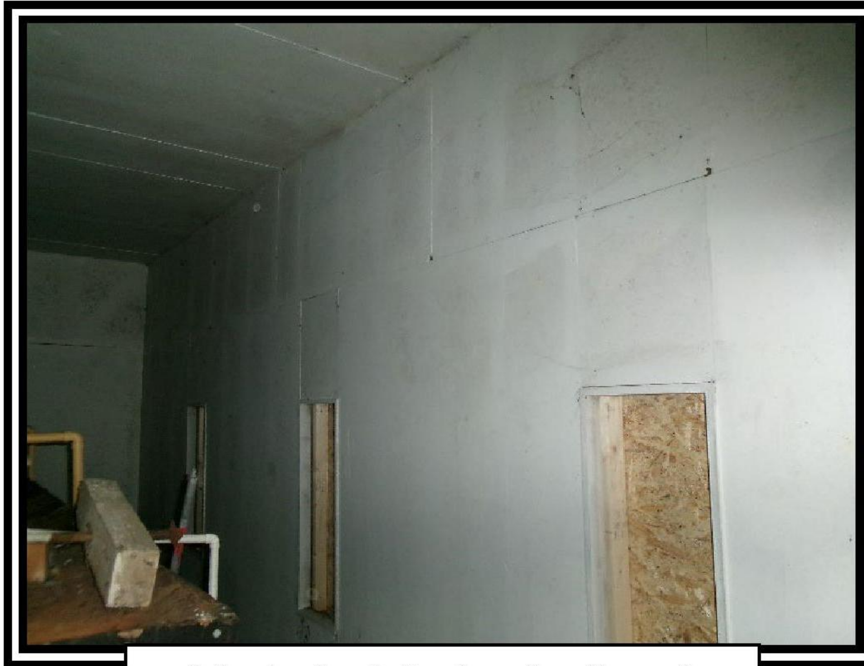
Asbestos insulating board wall panels
