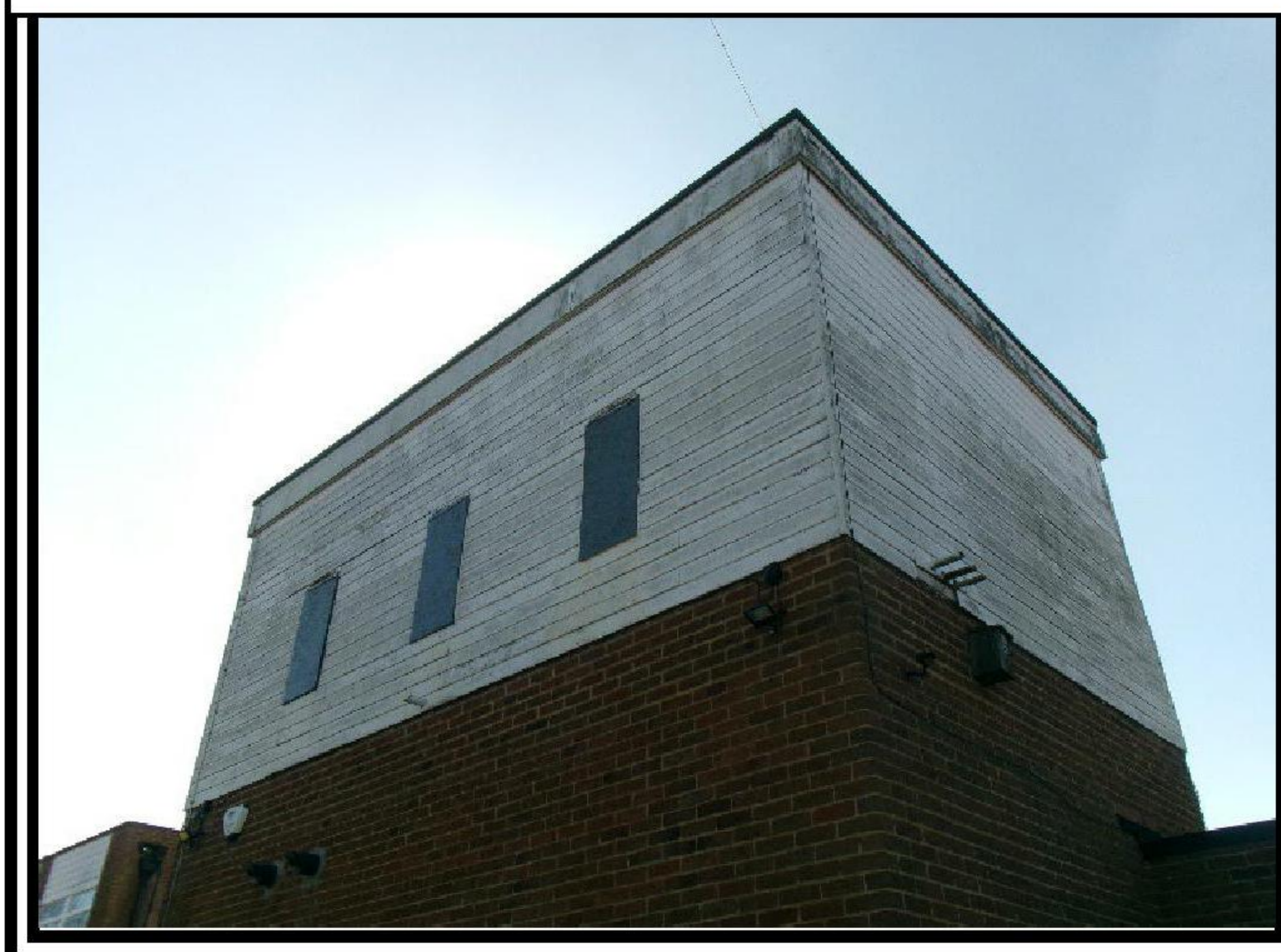
Asbestos cement shiplap panels to 072 Tank Room
