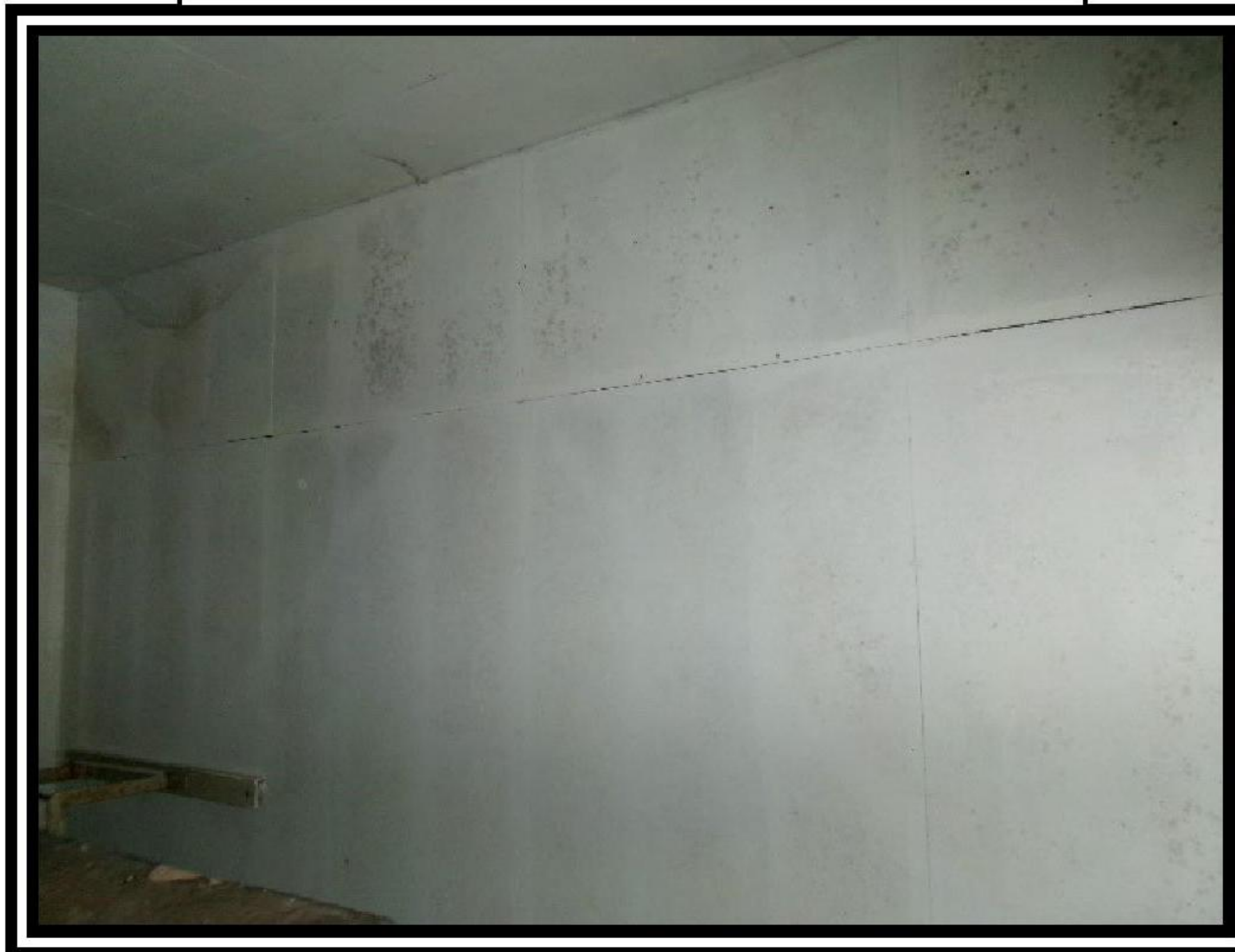
Asbestos insulating board wall panels
