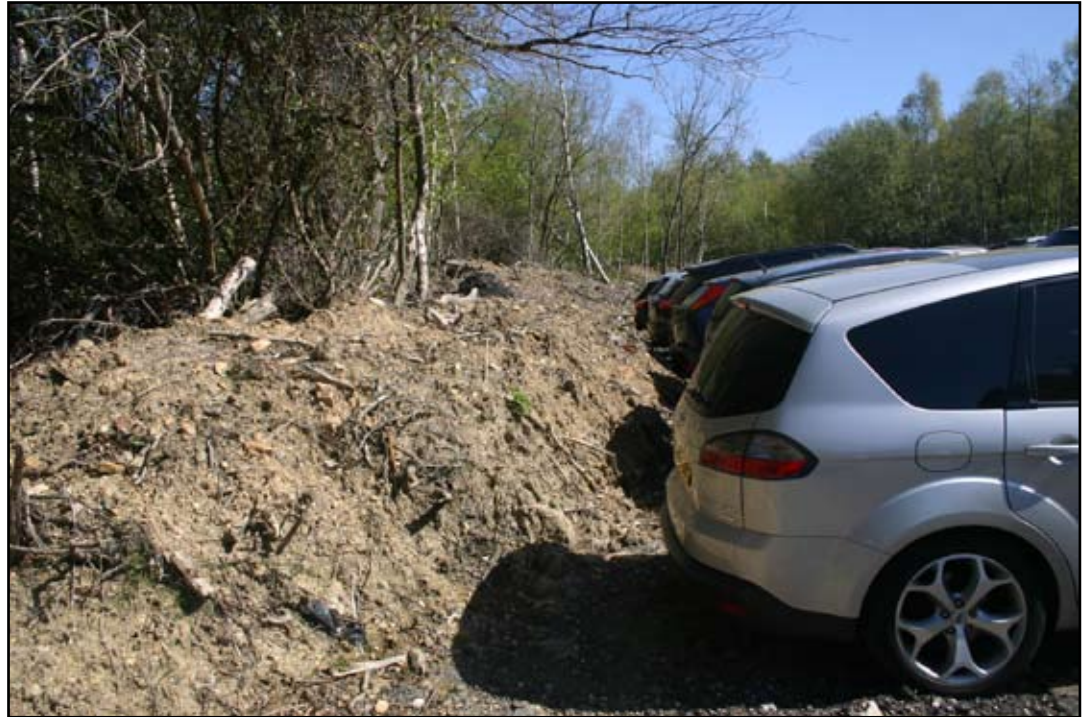
Some areas of cleared ground around the boundary of the car park have been formed into bunds. The bunds act as an interface between the woodland and hard core.
