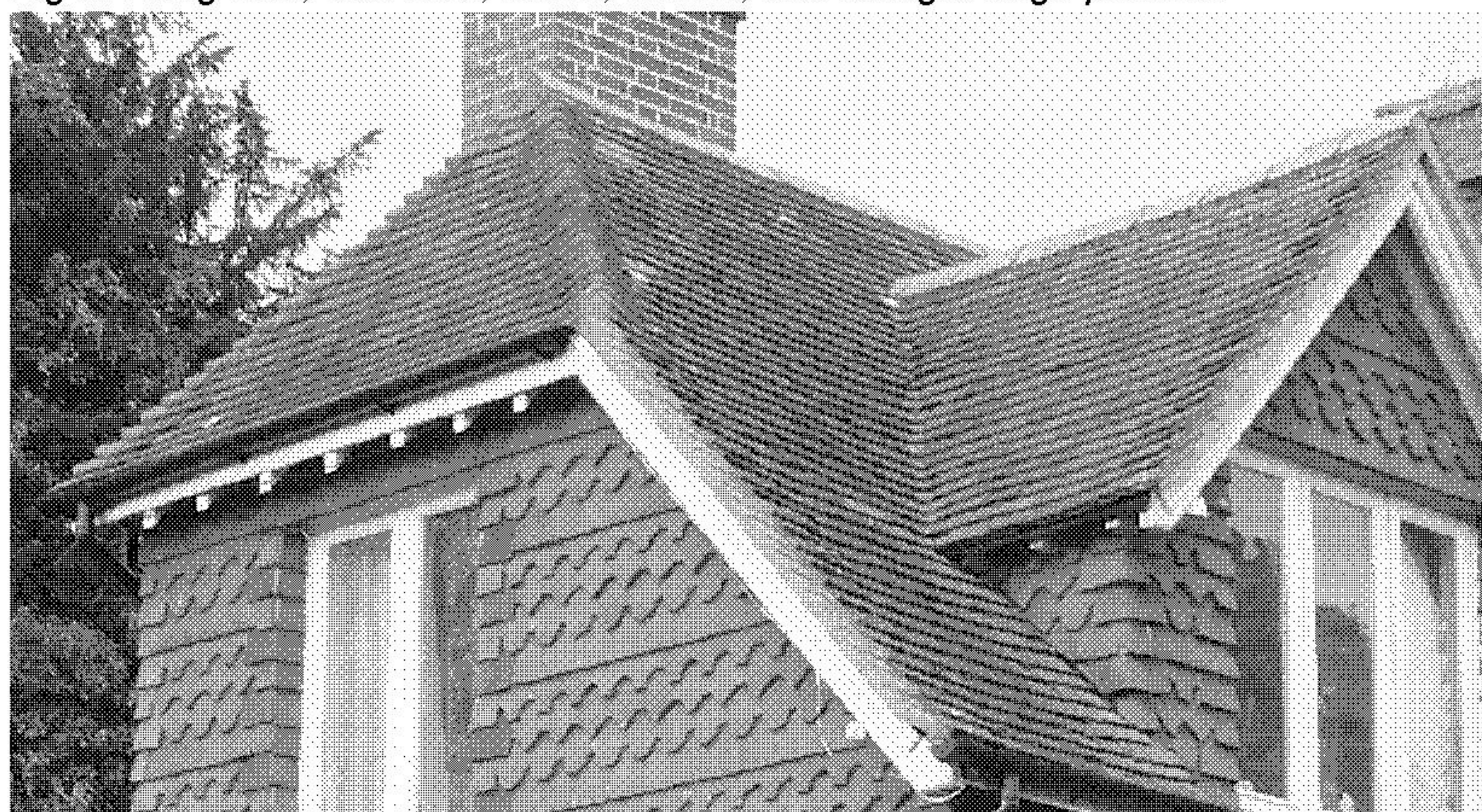
Fig 4: Darker plain roof tiles, with hogsback ridge tiles, and bonnet hips to the hipped end.
