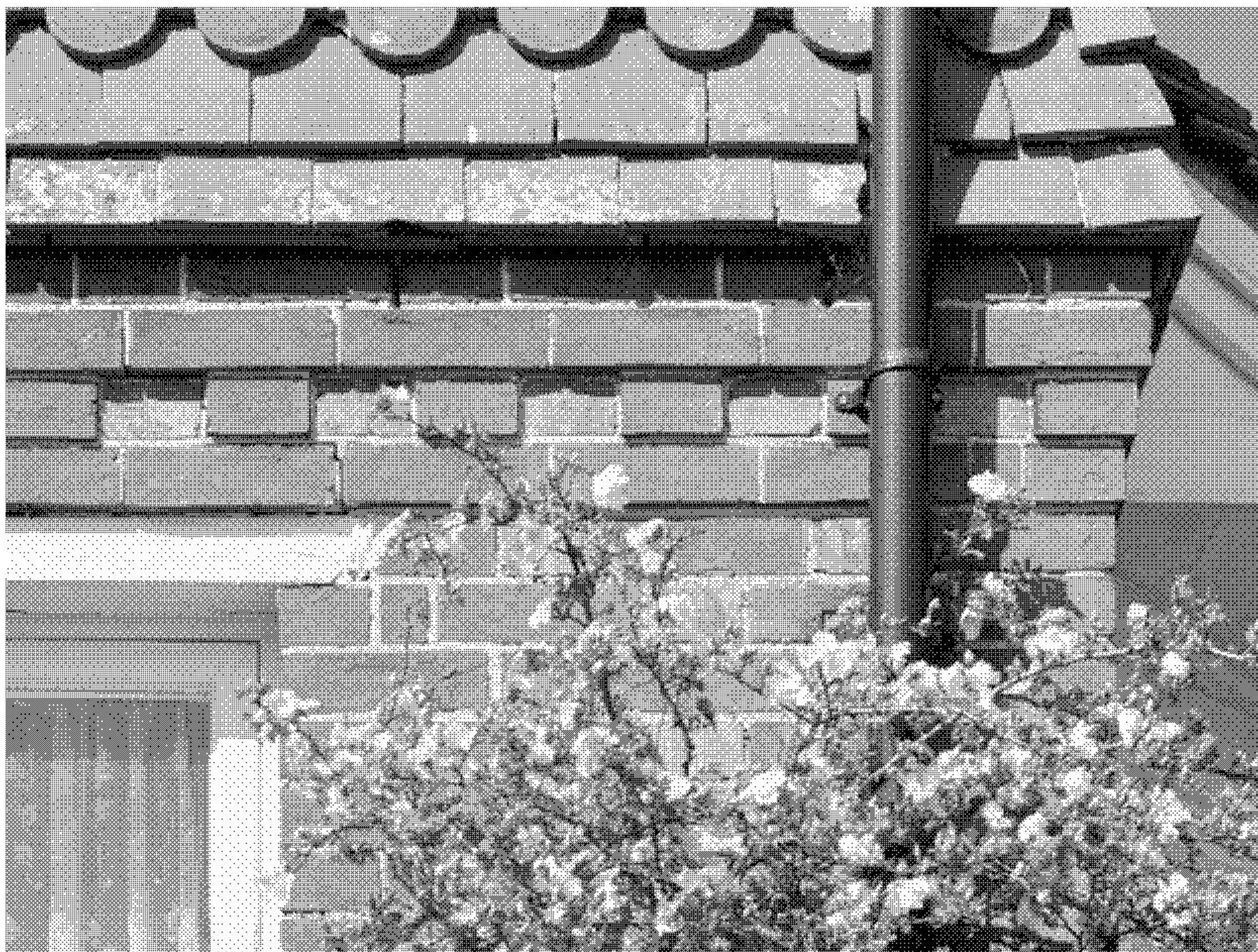
Fig 1: South-east corner, brickwork dentil.
