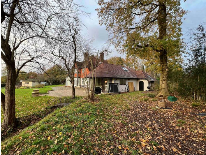
Rear elevation of White Lodge
