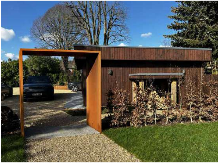
Ornamental garden arch in Corten steel at entrance to garden
