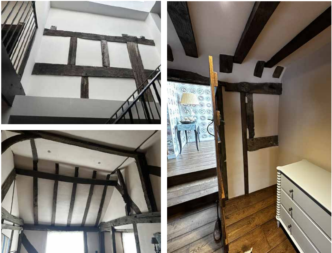
Photographs of restored historic oak frame
