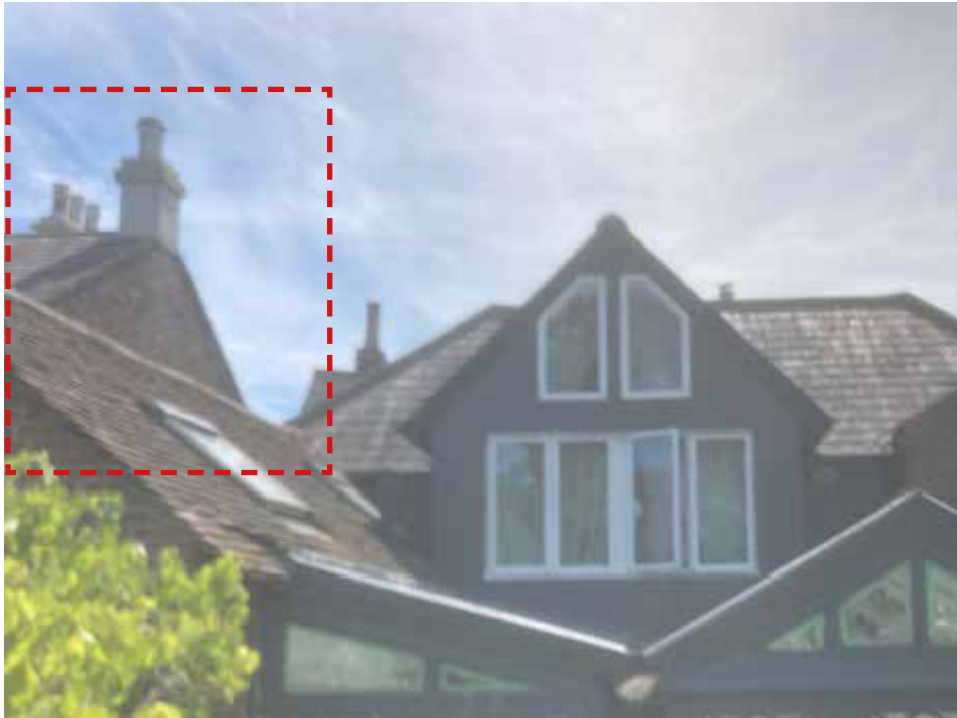
109 High Street south gable wall before re-rendering
