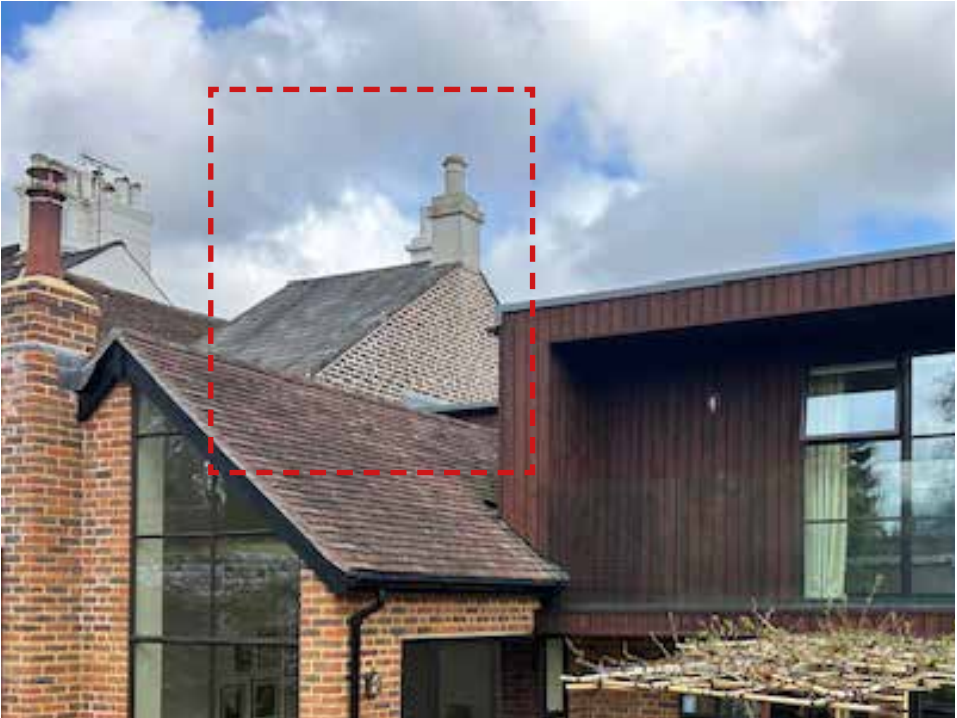
109 High Street south gable wall re-pointed in lime mortar
