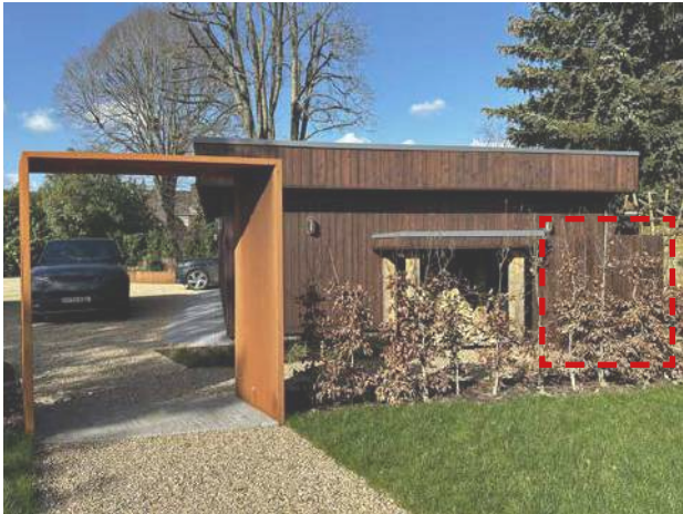
Recent photographs of the irrigation tank enclosure
