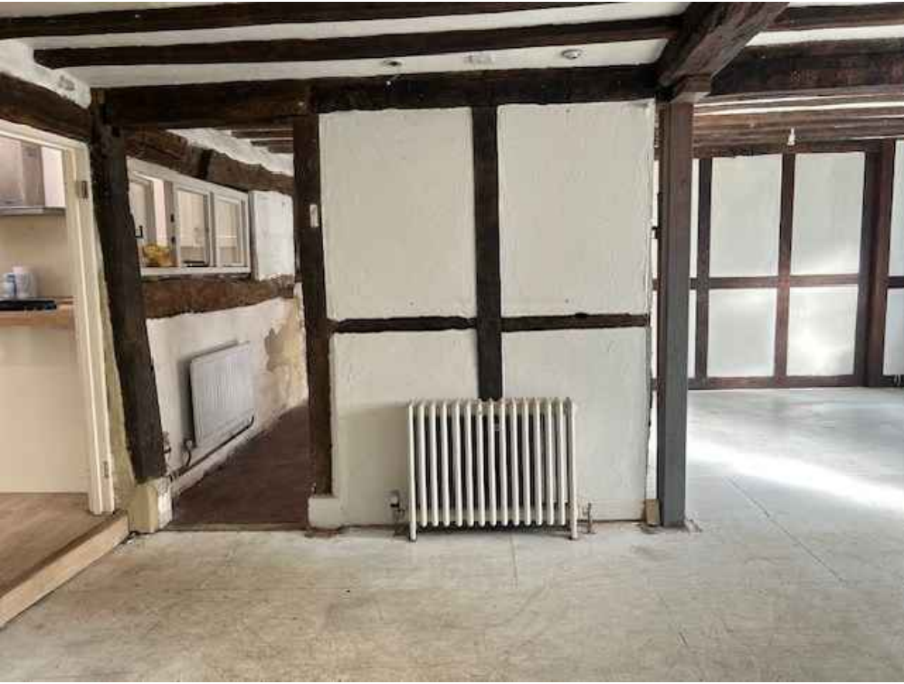
Partition wall in the lounge before removal
