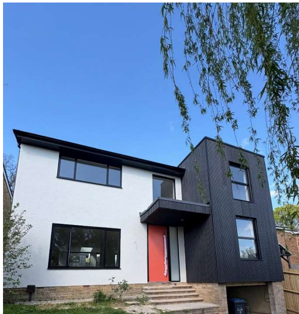
Above: Front facade taken from the front garden.
