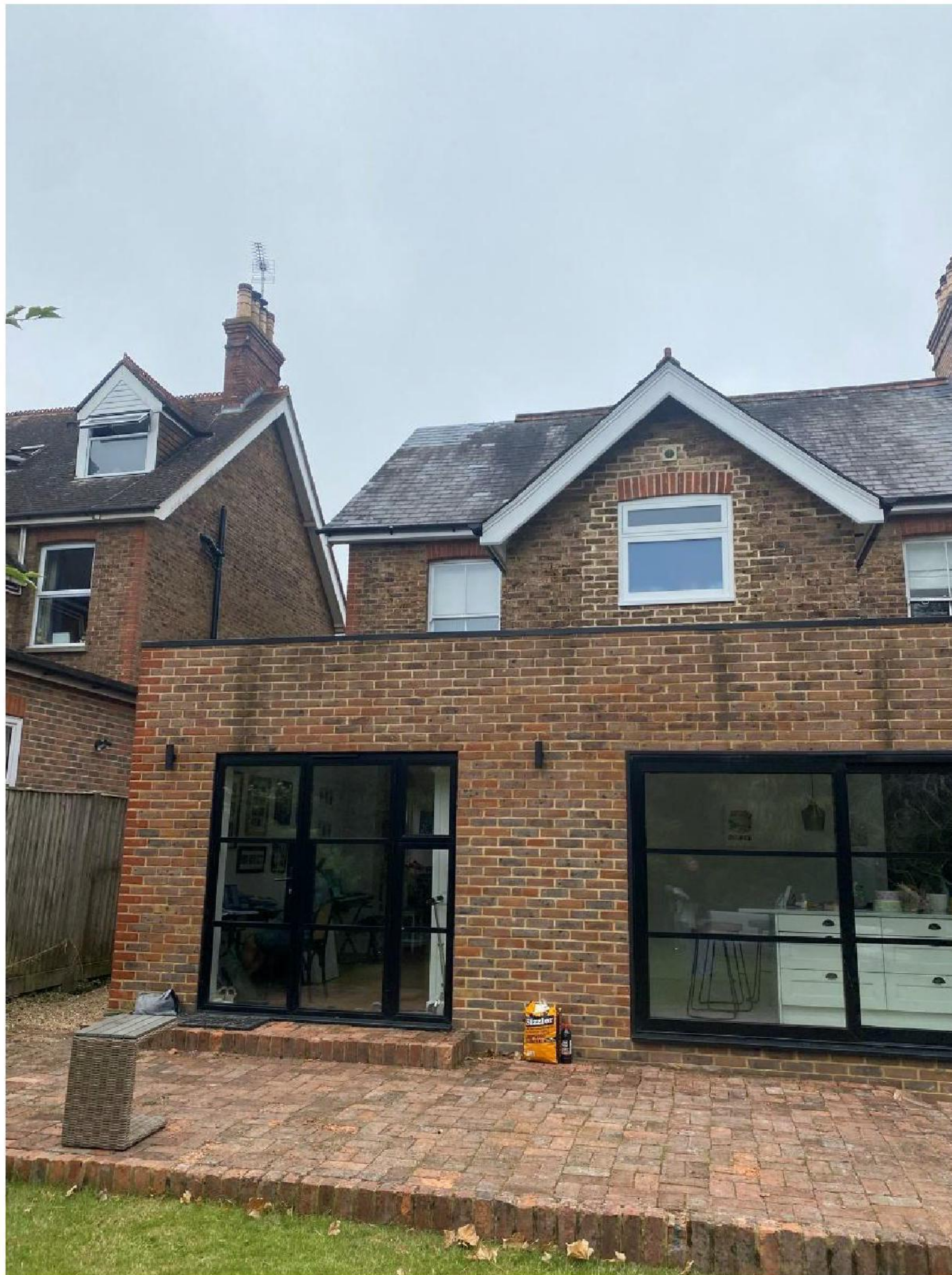
Photograph showing the rear of the application site and dormer of neighbouring property (no.16).
