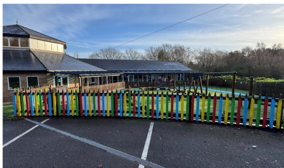
View to front of classroom Right hand side South East corner to be extended above
