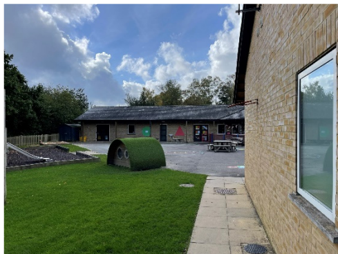
View to rear of classroom on Left hand side to be extended above
