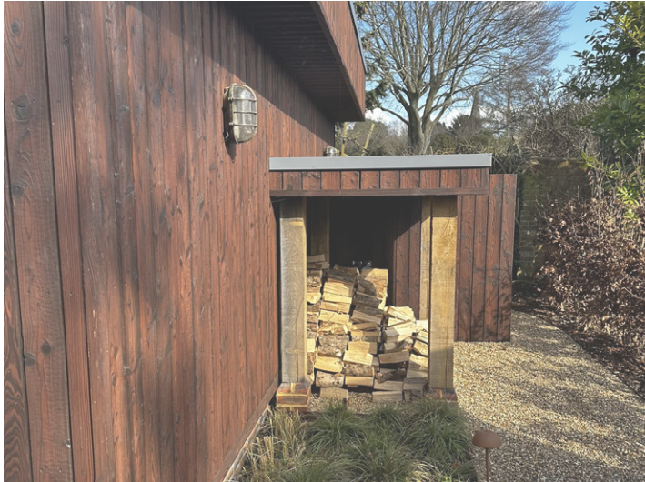
Current photograph- garage
