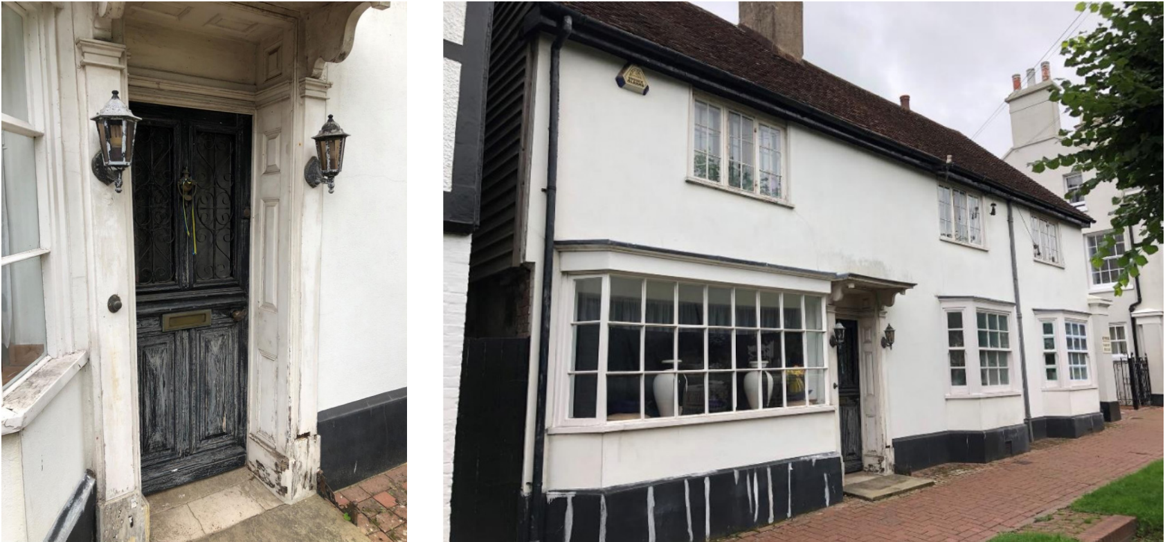
Photographs of front elevation before restoration works
