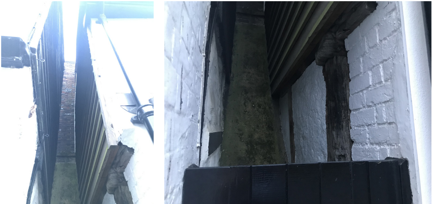
Recent photographs of timber weatherboarding
