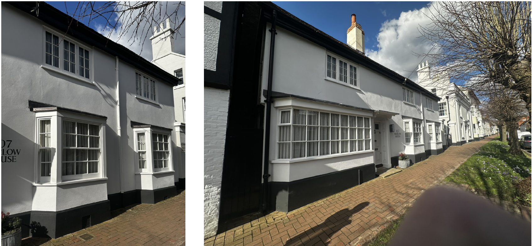
Photographs of front elevation after restoration works
