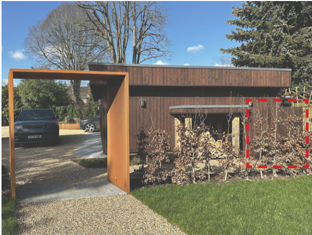
Recent photographs of the irrigation tank enclosure
