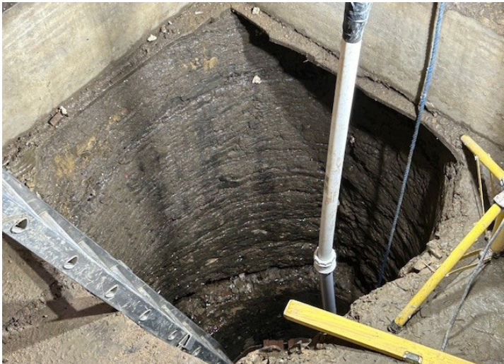
Opened well shaft
