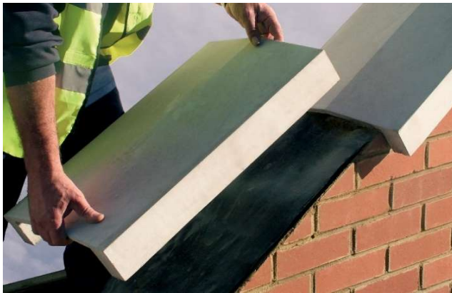
Parapet detailing – reconstituted stone
