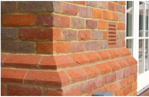
Plinth detailing – double kick
