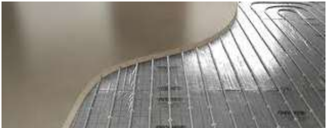
Under floor heating
