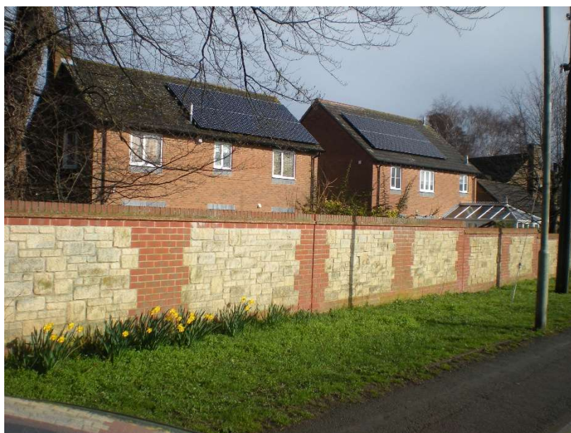
Figures 4: Solar PV installations on new build houses
