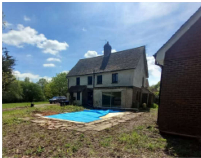
Figure 8: Existing dwelling on site to be demolished
