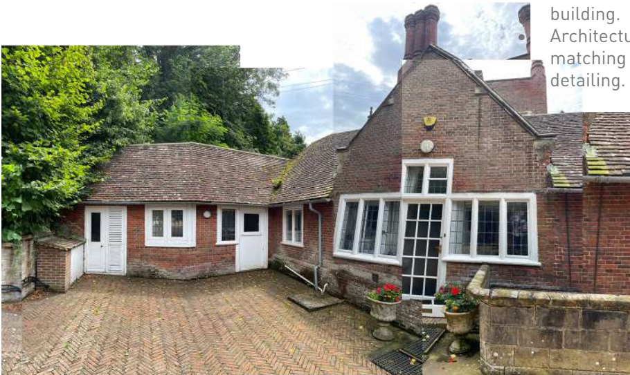
A1 - External view of services courtyard
