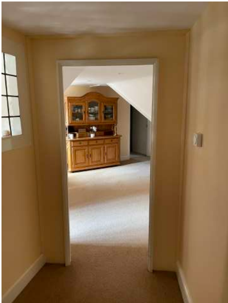
M Wall (right) to be removed
