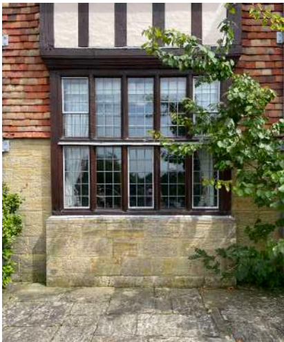
A2 - External and internal view of windows to library
