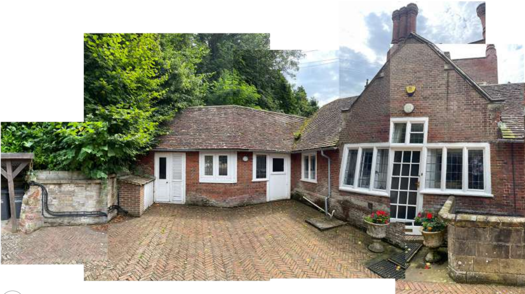
(A1) External view of gym and utility to be removed/extended
