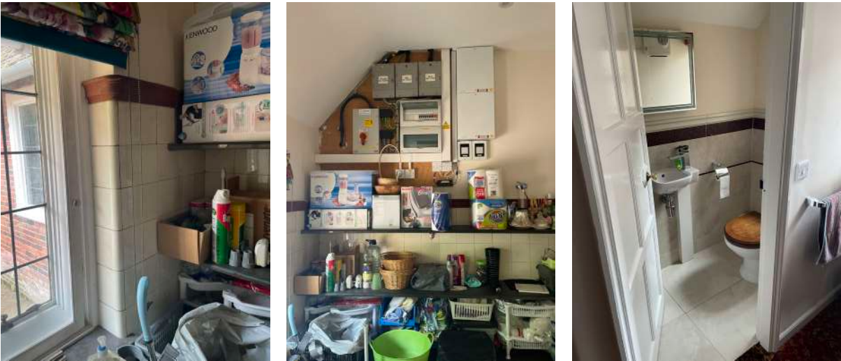
(A3) Internal views of utility to be removed
