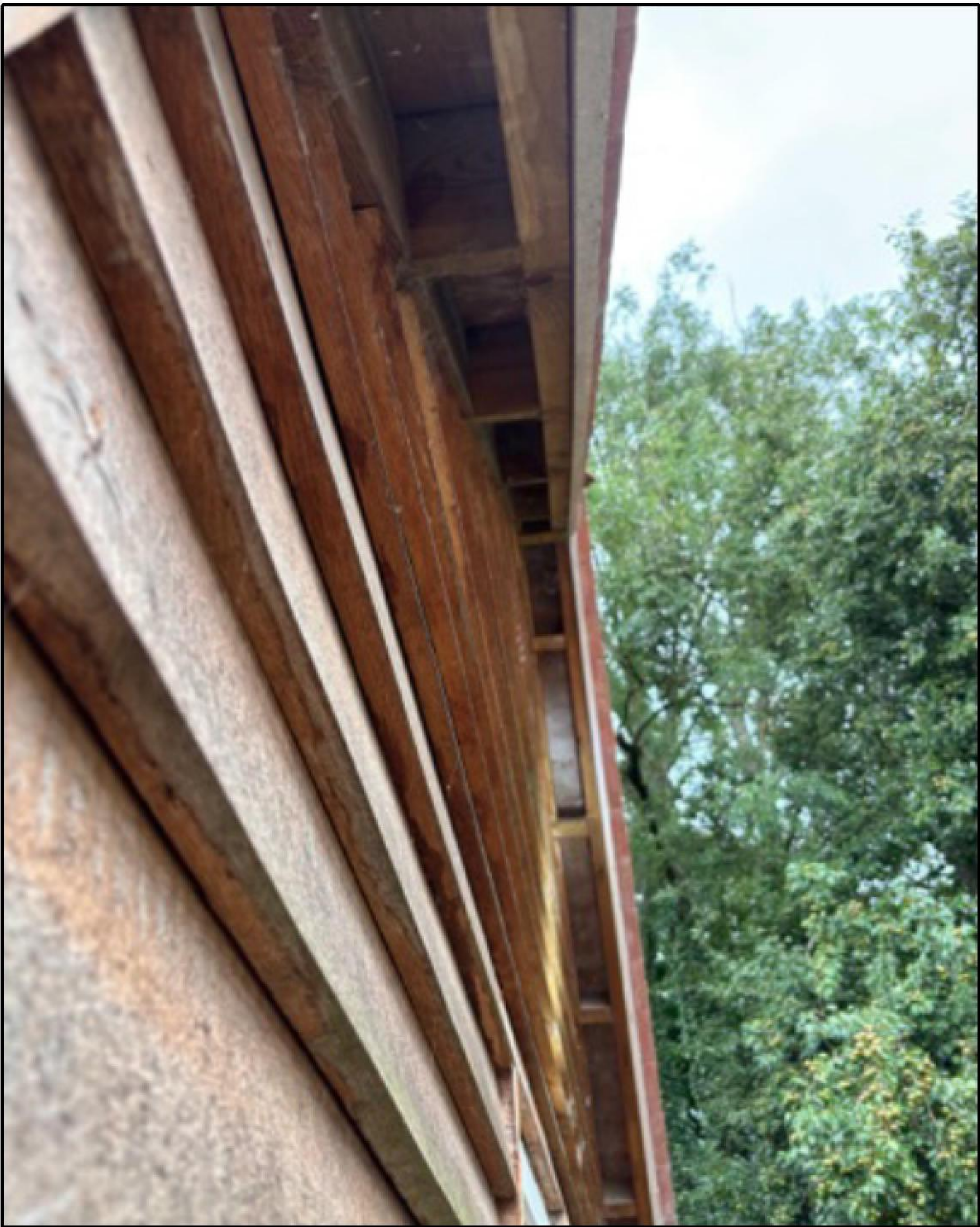
Photograph 11. An example of the tightly sealed cladding found on all elevations of the Visitor Reception building.
