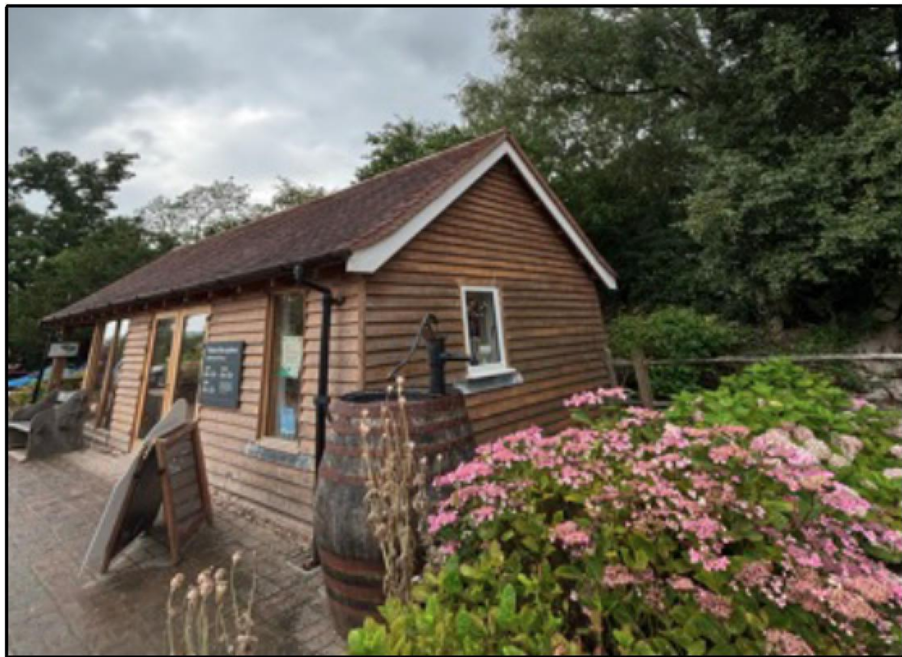
Photograph 1. An overview of the Visitor Reception building looking south-west.
