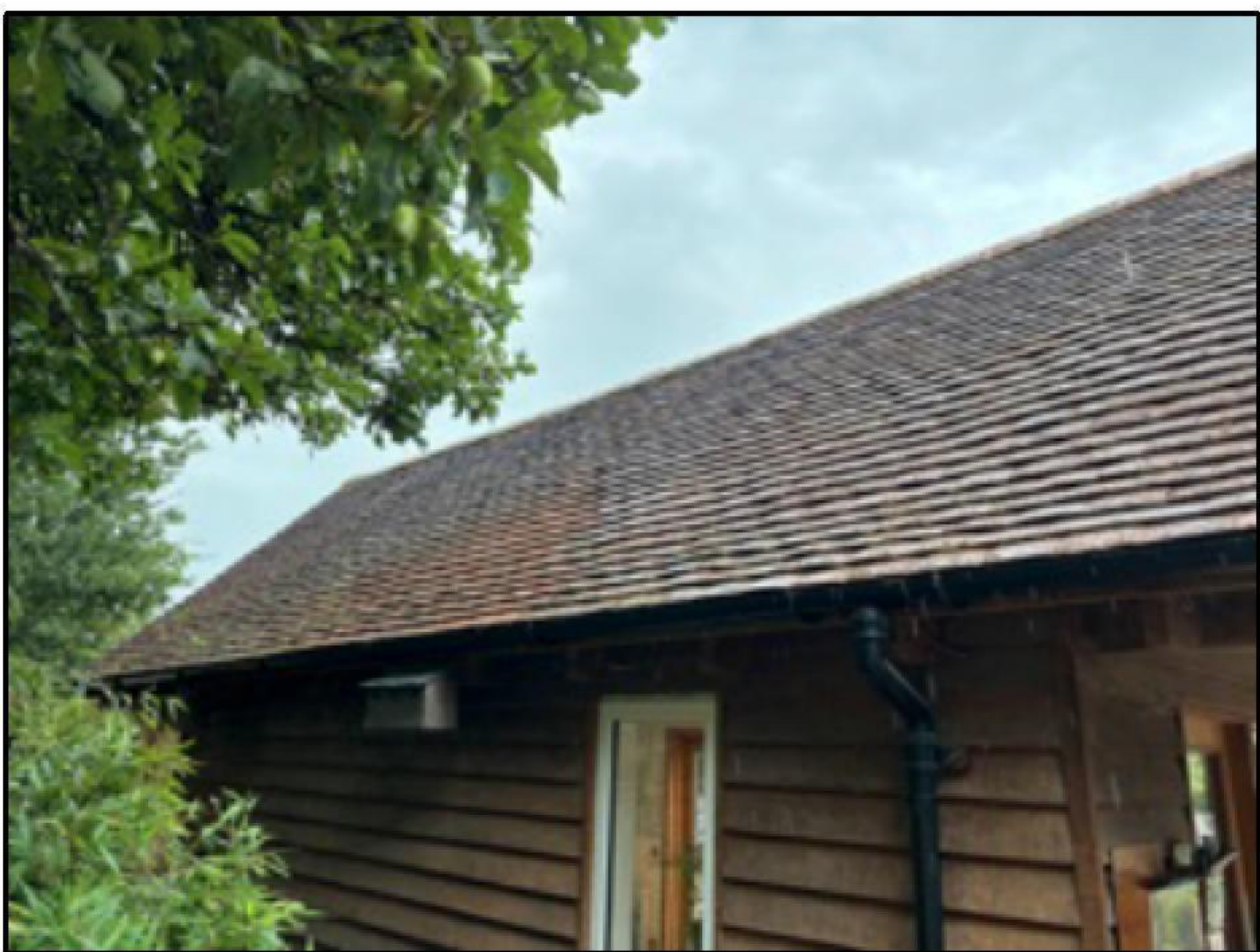
Photograph 10. The tightly sealed roof tiles on the rear (western elevation) of the Visitor Reception building
