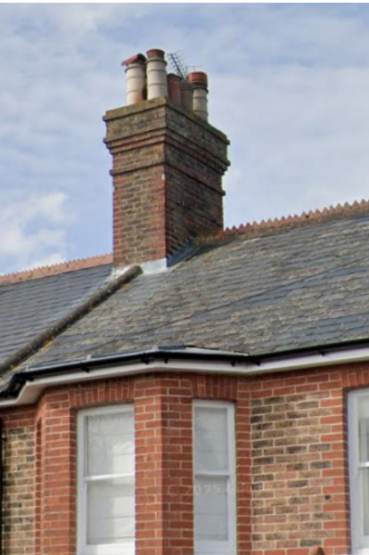
Larger scale chimneys seen on 1-8 Lewis Rd showing more decorative brick detailing, traditional flashing and chimney pots
