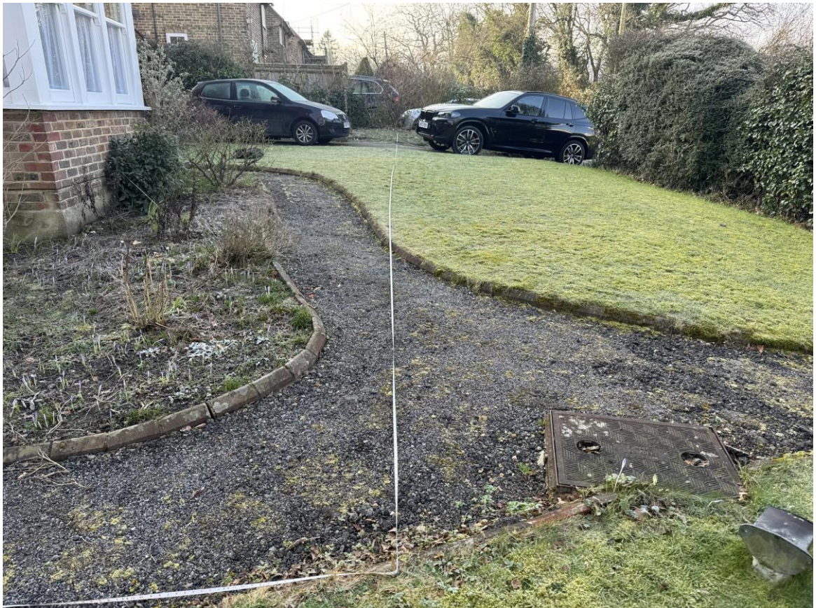
Image 3 shows the longer section with barrier extended across the driveway
