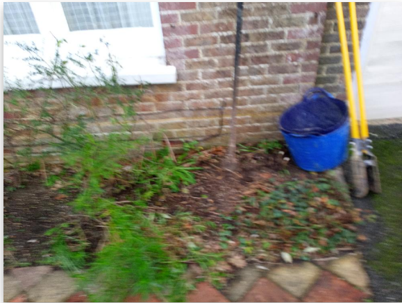
Fig 1.1: Trial Hole Location
