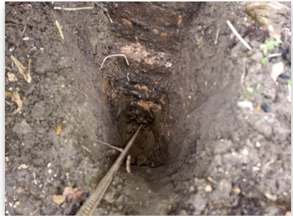
Fig 1.2: Trial Hole Footing
